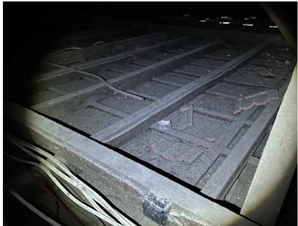
Line ID 31: Internal, GF, Cessnock House, East Wing, Ceiling Space, Dust - Lead Detected (990 mg/kg)
