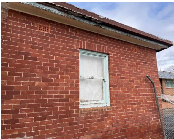
Line ID 21.1: External, GF, All Areas, Windows & frames, Throughout, Blue (Light) Paint - Lead Detected (2.4% w/w)
