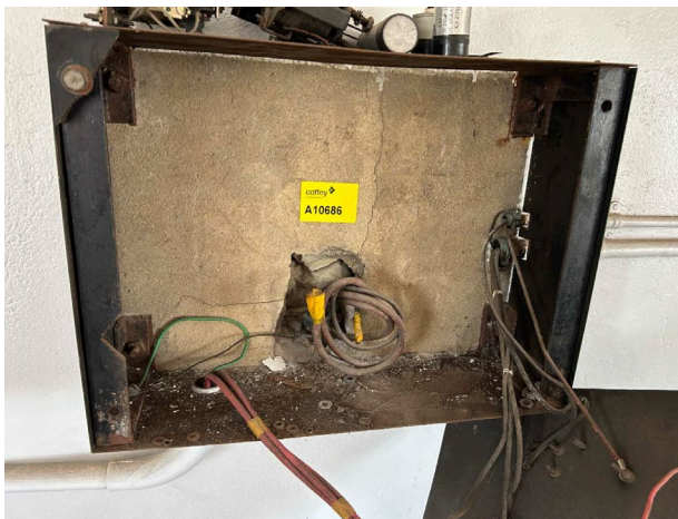
Line ID 103: Internal, L2, Lift Motor Room, Electrical Cabinet, Dust - Chrysotile Asbestos Detected
