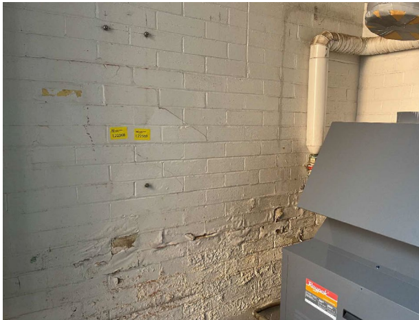
Line ID 113: Internal, GF, Central Wing, Day Surgery/Recovery, Plant Room, Walls, White Paint - Lead Detected (0.099% w/w)
