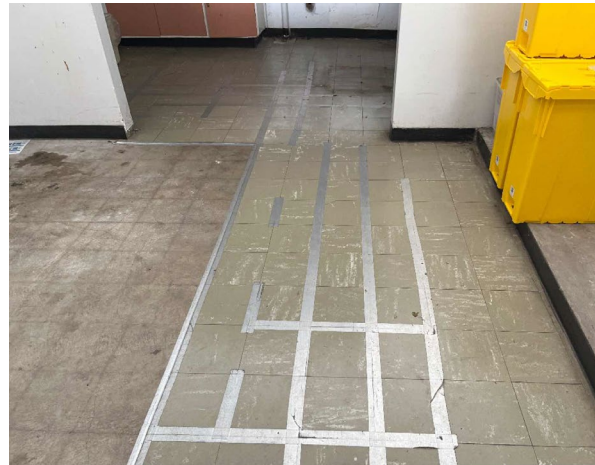
Line ID 18: Internal, GF, Laundry, Floor covering, Throughout, Vinyl Floor Tiles (grey with white specs) - Suspected Asbestos
