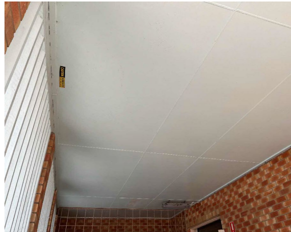
Line ID 1.1: External, GF, Mortuary, All Areas, Awning, Entrance, Fibre Cement Sheeting - Chrysotile Asbestos Detected
