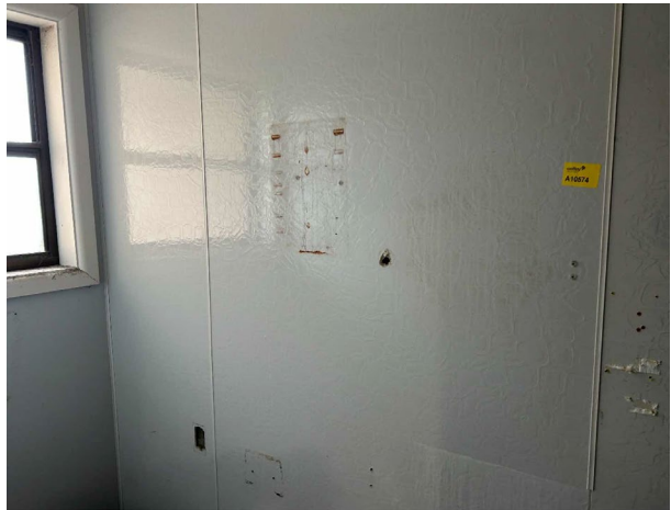
Line ID 19: Internal, GF, Cessnock House, West Wing, Comms Cupboard 0017, Walls, Fibre Cement Sheeting - No Asbestos Detected
