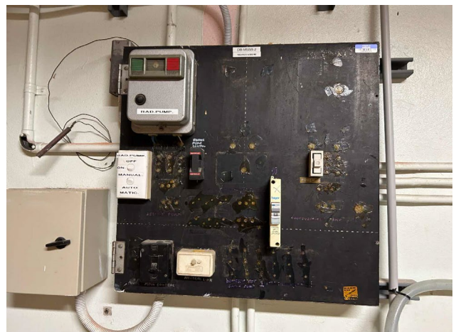
Line ID 53: Internal, GF, Central Wing, North Section, Plant Room 1073, Electrical Switch Board, Bituminous Backing Board - Suspected Asbestos
