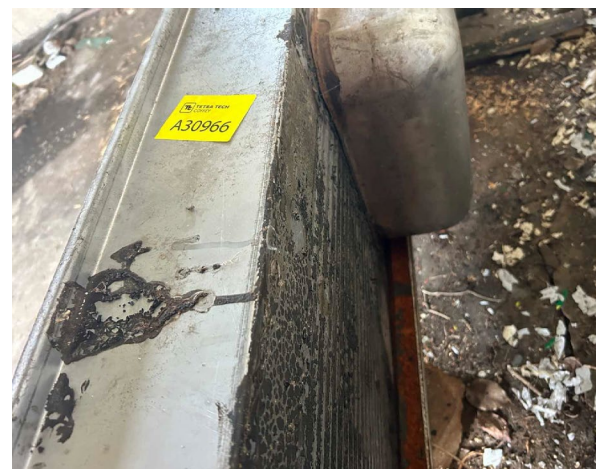
Line ID 15: Internal, GF, Old Mortuary, North Room, to Redundant Sink, Bituminous Material - No Asbestos Detected
