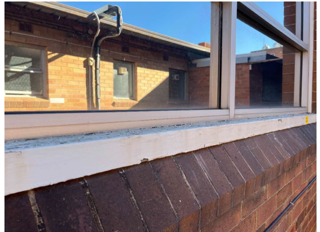
Line ID 108: External, GF, Central Wing, Northern Courtyard, Timber Window Frames, White Paint - Lead Detected (1.8% w/w)
