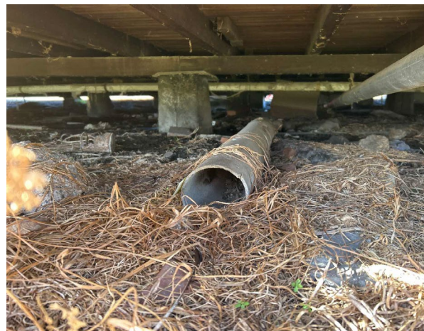
Line ID 9: External, GF, Workshops, All Areas, Central Section, Subfloor, Pipework, Moulded Fibre Cement - Chrysotile and Amosite Asbestos Detected
