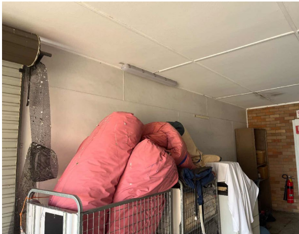
Line ID 43: Internal, GF, Palliative Care Storage Loading Dock, Wall lining, Throughout, Fibre Cement Sheetting - No Asbestos Detected
