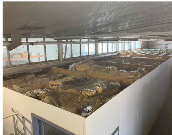
Line ID 62: Internal, GF, Laundry, Insulation Batts, On Top of Office Ceiling, Insulation Material - Suspected SMF
