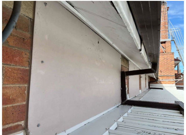
Line ID 33: External, Roof, ED Wing, Eaves, Throughout, Fibre Cement Sheeting - No Asbestos Detected
