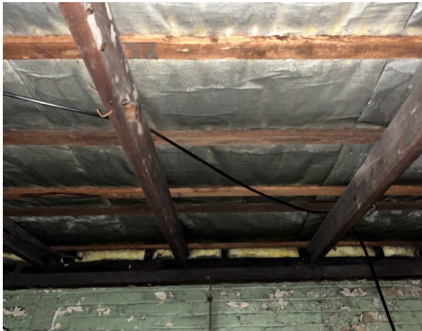
Line ID 59: Internal, GF, 1044, Painters Room, Ceiling Space, Sarking, Insulation Material - Suspected SMF
