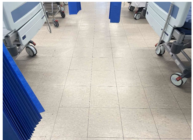
Line ID 40: Internal, GF, Central Wing, Day Surgery/Recovery, Floor covering, Throughout, Vinyl Floor Tiles (white with grey specks) - Chrysotile Asbestos Detected
