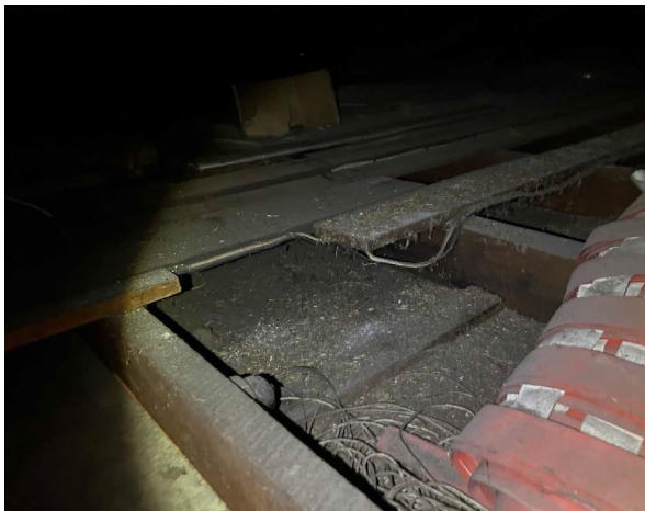
Line ID 18: Internal, GF, Workshops, Central Section, Ceiling Space, Dust - Chrysotile Asbestos Detected
