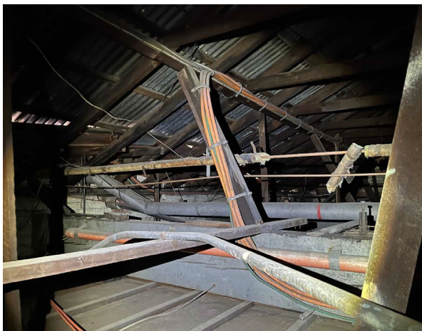
Line ID 64: Internal, GF, Main Workshop Area, Ceiling Space, Pipework, Central, Insulation Material - Suspected SMF
