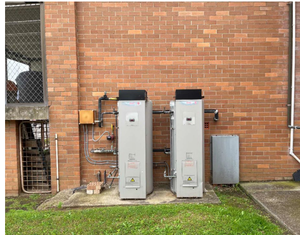
Line ID 23: External, GF, All Areas, Hot Water Heater, Adjacent Roof Access, Insulation Material - Suspected SMF
