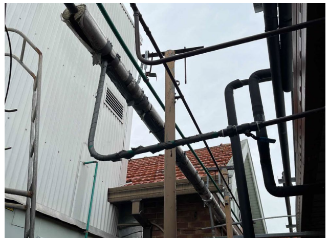
Line ID 133: External, GF, Central Wing, Central Courtyard, Pipework, Central, Insulation Material - Suspected SMF
