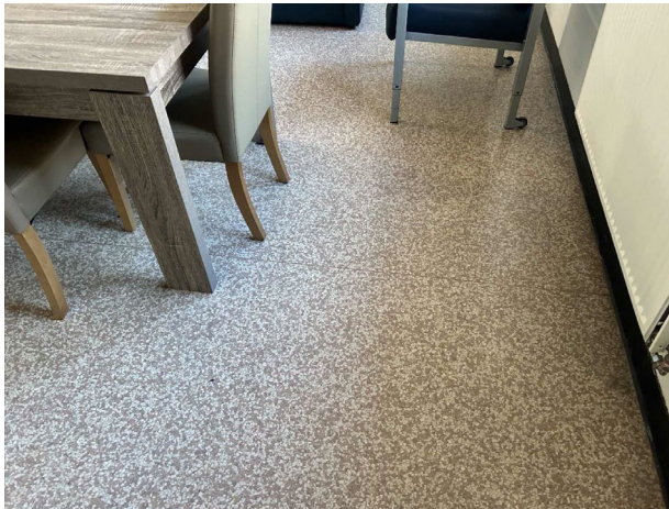
Line ID 70: Internal, GF, Central Wing, Ward A, Staff Room 1118, Floor Covering, Fibrous Backed Vinyl Sheet - No Asbestos Detected
