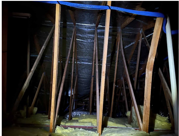
Line ID 37: Internal, GF, Cessnock House, West Wing - Ceiling Space, Roof Lining, Sarking Insulation - Suspected SMF
