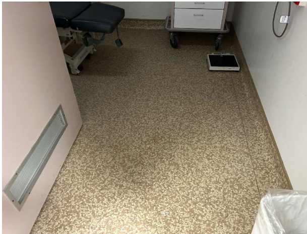
Line ID 61: Internal, GF, Central Wing, North Section, Room 1033, Floor Covering, Fibrous Backed Vinyl Sheet - No Asbestos Detected
