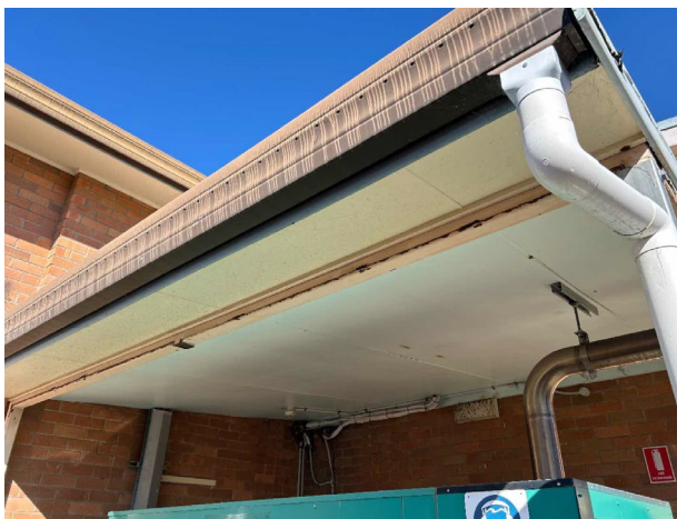
Line ID 10: External, GF, Central Wing, Northern Generator Awning, Fibre Cement Sheetting - No Asbestos Detected
