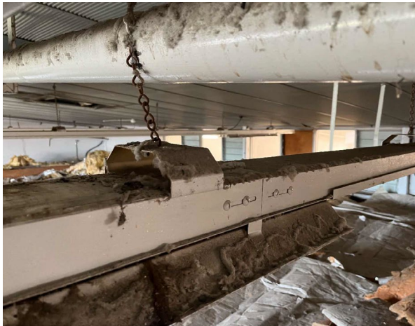
Line ID 54: Internal, GF, All Areas, Laundry, High Level Surfaces, Throughout, Dust - Lead Detected (270 mg/kg)
