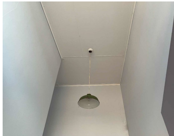
Line ID 45: Internal, GF, Room 1032, Toilet, Ceiling, Throughout, Fibre Cement Sheet - Chrysotile and Amosite Asbestos Detected
