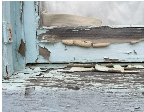
Line ID 21: External, GF, All Areas, Windows & frames, Throughout, Blue (Light) Paint - Lead Detected (2.4% w/w)
