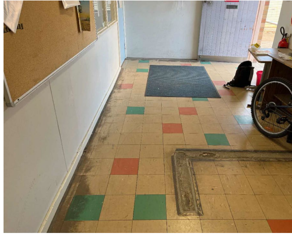
Line ID 5: Internal, GF, Storeroom, Main Foyer & Offices, Throughout, Vinyl Floor Tiles (cream with white specs) - Chrysotile Asbestos Detected
