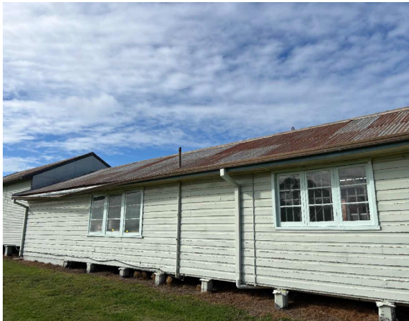
Line ID 35: External, GF, Workshops, All Areas, All Sections, Roof and Metal Work, Brown Paint - Lead Detected (0.26% w/w)
