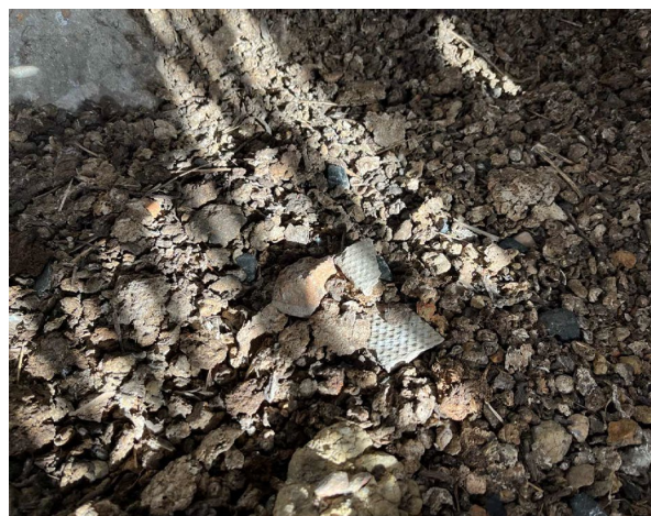
Line ID 10.1: External, GF, Room 1040, Old Coal Bunker, Floor, Throughout, Fibre Cement Debris - Chrysotile, Amosite and Crocidolite Asbestos Detected
