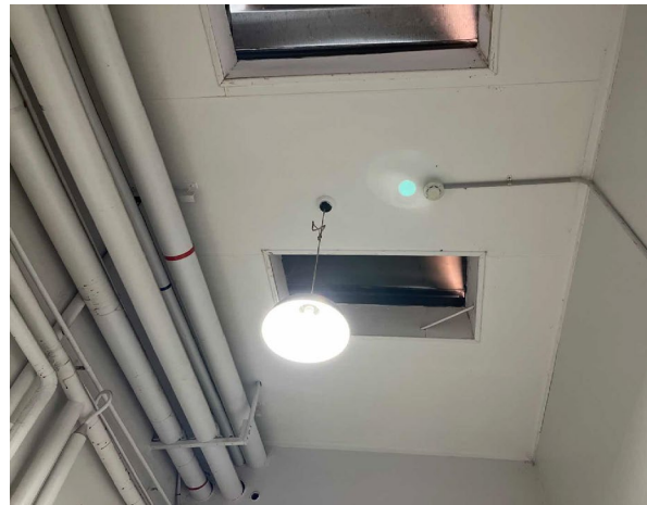
Line ID 44: Internal, GF, Room 1021 & 1022, Ceiling Lining, Throughout, Fibre Cement Sheetting - Chrysotile and Amosite Asbestos Detected
