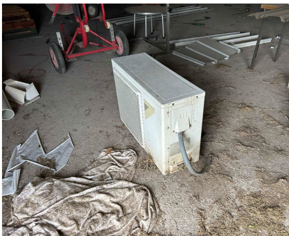
Line ID 46: Internal, Basement, Storage Area, Adjacent Entrance, Redundant AC Unit, R22 Hydrochlorofluorocarbon (HCFC) - ODS Refrigerant
