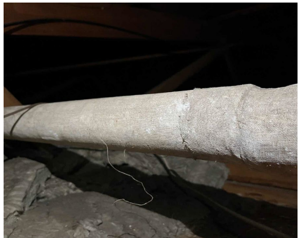
Line ID 9.1: Internal, GF, Storeroom Ceiling Space, Pipework, Throughout, Lagging - Amosite Asbestos Detected
