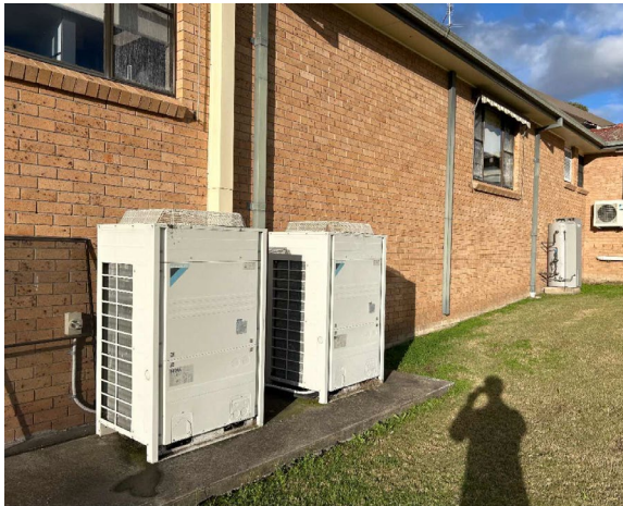
Line ID 44: External, GF, Cessnock House, West Wing, South, AC Units, R410A Hydrofluorocarbon (HFC) - Non ODS Refrigerant
