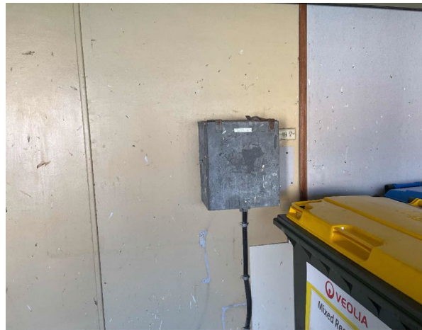
Line ID 23.1: Internal, GF, Workshops, Northern Section, Electrical Distribution Board 19 - Incinerator, Compressed Bituminous Panel - Suspected Asbestos
