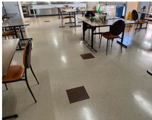
Line ID 10: Internal, GF, Kitchen, Cafeteria Floor Covering, Various Throughout, Vinyl Floor Tiles (brown) - Chrysotile Asbestos Detected
