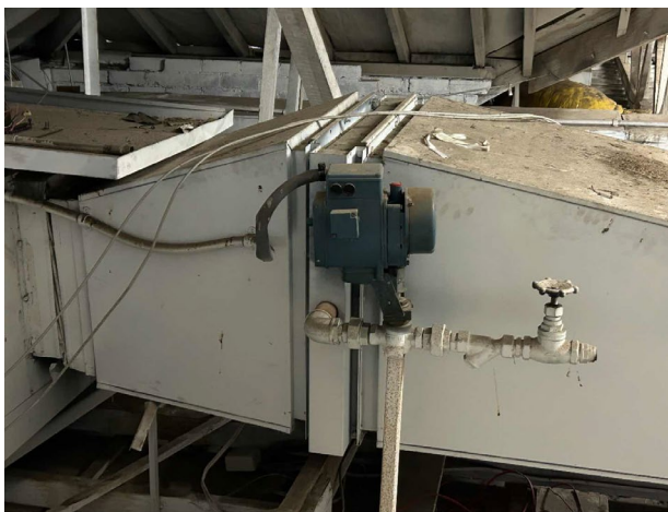
Line ID 36: Internal, GF, All Areas, Ceiling Space, Various Throughout, Heater Banks to AC Ducting, Internal Lining, Millboard Insulation - Suspected Asbestos
