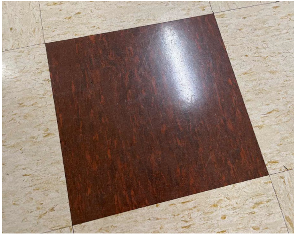
Line ID 10.1: Internal, GF, Kitchen, Cafeteria Floor Covering, Various Throughout, Vinyl Floor Tiles (brown) - Chrysotile Asbestos Detected
