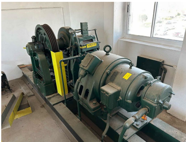
Line ID 120: Internal, L2, Lift Motor Room, Lift Motor, Green Paint - Lead Detected (2.1 % w/w)
