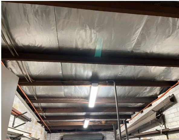
Line ID 68: Internal, GF, Room 1034, Storage, Sarking, Roof Lining, Insulation Material - Suspected SMF
