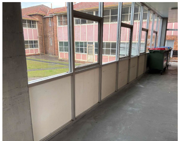
Line ID 4.1: External, GF, All Areas, Infill Panels, Below Windows, Fibre Cement Sheet - Chrysotile Asbestos Detected
