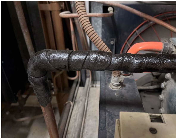
Line ID 19.1: Internal, Basement, Switchboard Room, 0003, Plant & Equipment Pipework, Central, Bituminous Wrap - No Asbestos Detected
