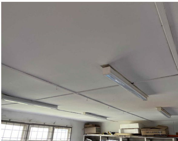
Line ID 44.1: Internal, GF, Workshops, Central Section, Wall & Ceiling Lining, Blue (Light) Paint - Lead Detected (0.25% w/w)
