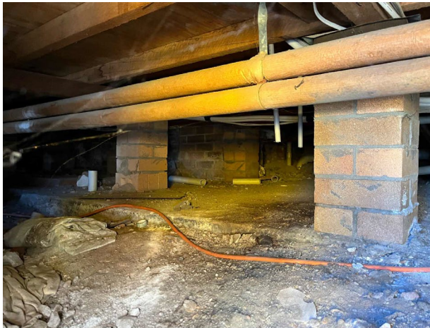
Line ID 151: Internal, GF, Central Wing, North Section, Sub-Floor Area, Pipework, Insulation Material - Suspected SMF
