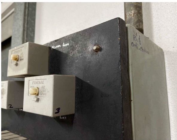
Line ID 17.1: Internal, Basement, Switchboard Room, 0003, Electrical Distribution Board, Southwest, Compressed Bituminous Panel - Suspected Asbestos
