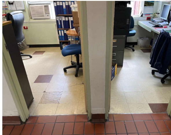
Line ID 15: Internal, GF, Kitchen, Rooms 1008 & 1007, Various Throughout, Vinyl Floor Tiles (brown) - Chrysotile Asbestos Detected
