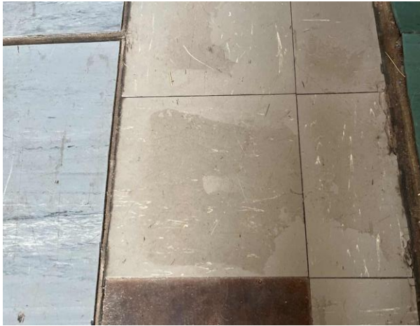
Line ID 14: Internal, GF, Dining/Laundry, Floor Covering, Various Throughout, Vinyl Floor Tiles - Chrysotile Asbestos Detected
