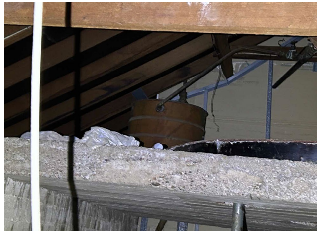
Line ID 160: Internal, L1, Southeast Wing, Ceiling Space, North, Old Metal Water Tank, Insulation Material - Suspected SMF
