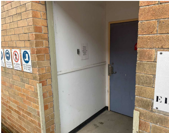
Line ID 12: External, GF, Workshop Entrance, Wall Lining, Fibre Cement Sheeting - Chrysotile Asbestos Detected
