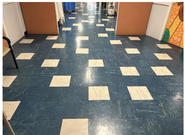
Line ID 74: Internal, GF, Central Wing, Ward B, Floor covering, Various Throughout, Vinyl Floor Tiles (blue) - Chrysotile Asbestos Detected
