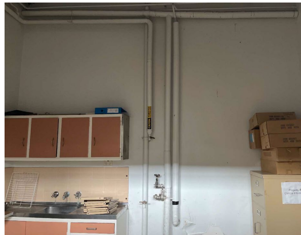
Line ID 27: Internal, GF, Laundry, Pipework, Throughout, Lagging - Amosite Asbestos Detected
