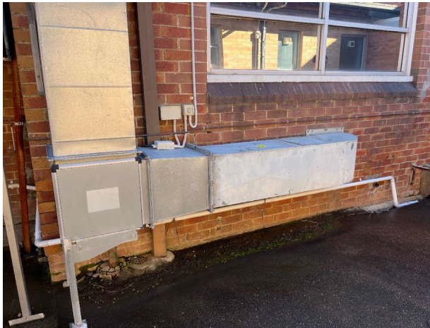
Line ID 107: External, GF, Central Wing, Northern Courtyard, Ductwork, Throughout, Grey (Light) Paint - Lead Detected (0.22% w/w)
