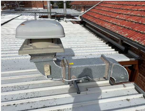
Line ID 28: External, Roof, Central Wing, North Section, Central Area, Ductwork Flange Joints, Mastic Sealant - No Asbestos Detected
