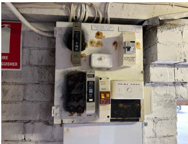
Line ID 87: Internal, GF, Southeast Wing, Southern Sub-Floor Area, Adjacent Entrance, Electrical Board, Bituminous Backing Board - Suspected Asbestos
