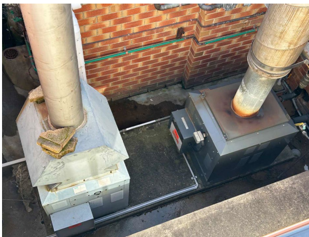
Line ID 132: External, GF, Central Wing, Central Courtyard, Boilers and Associated Pipework, Insulation Material - Suspected SMF
