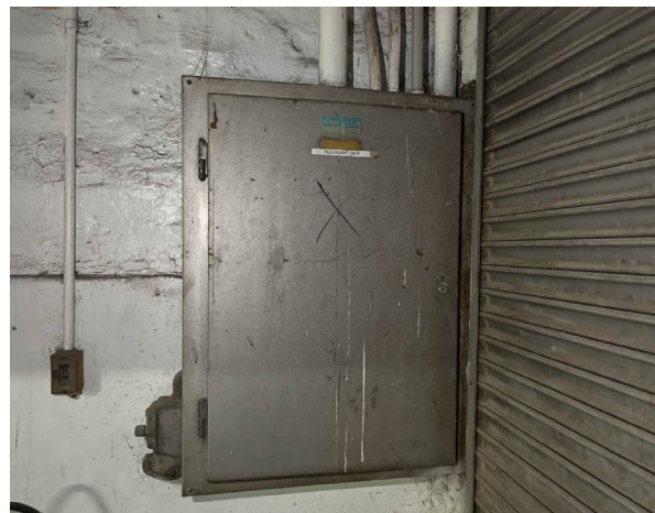
Line ID 14: Internal, GF, 1044, Painters Room, Electrical Distribution Board DB18, Adjacent Roller Door, Internal Electrical Components - Suspected Asbestos
