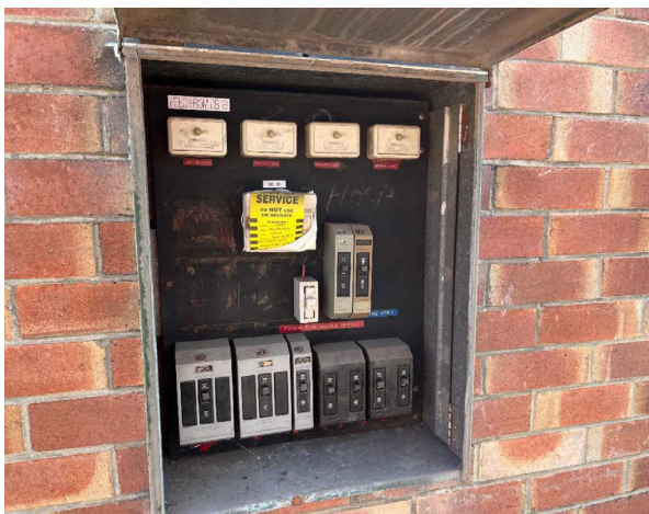
Line ID 3: External, GF, Storeroom Driveway, Electrical Distribution Board, Northern Boundary, Compressed Bituminous Panel - Suspected Asbestos
