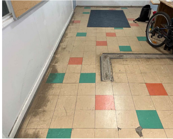
Line ID 6: Internal, GF, Storeroom, Main foyer & Offices, Various Throughout, Vinyl Floor Tiles (green) - Chrysotile Asbestos Detected
