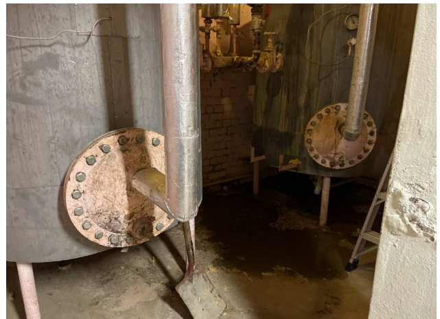
Line ID 51.1: Internal, GF, Central Wing, North Section, Plant Room 1073, Boiler, Large Gasket, Gasket Material - Chrysotile Asbestos Detected
