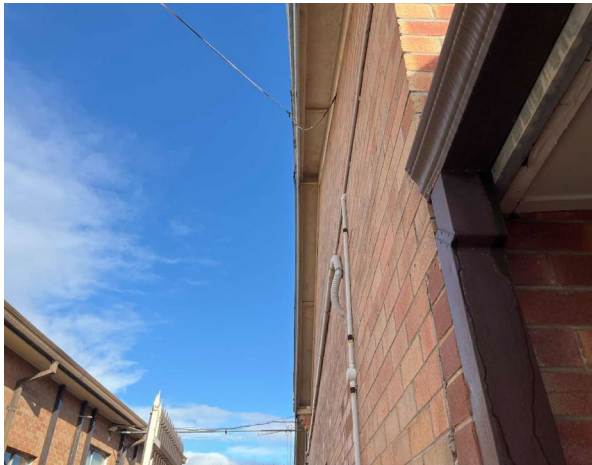
Line ID 2.1: External, GF, All Areas, Eaves, Throughout, Fibre Cement Sheetting - Chrysotile Asbestos Detected
