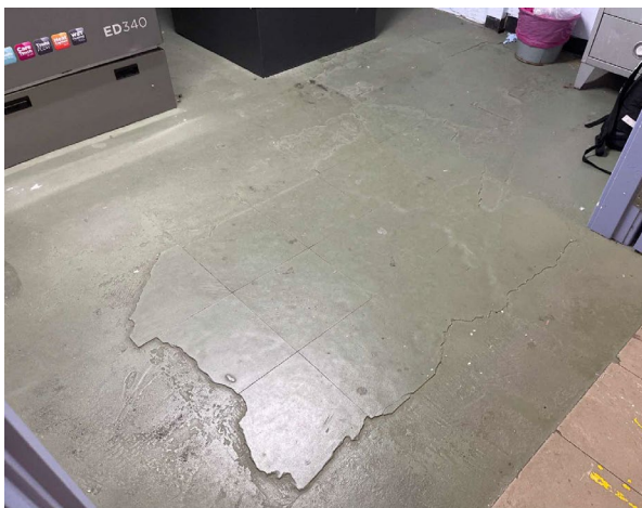
Line ID 20: Internal, GF, Laundry, Floor Covering, Throughout, Vinyl Floor Tiles (grey with white specs, large squares) - Painted green - Chrysotile Asbestos Detected
