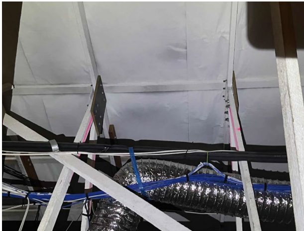
Line ID 145: Internal, GF, Central Wing, North Section, Ceiling Space, Sarking, Roof Lining, Insulation Material - Suspected SMF
