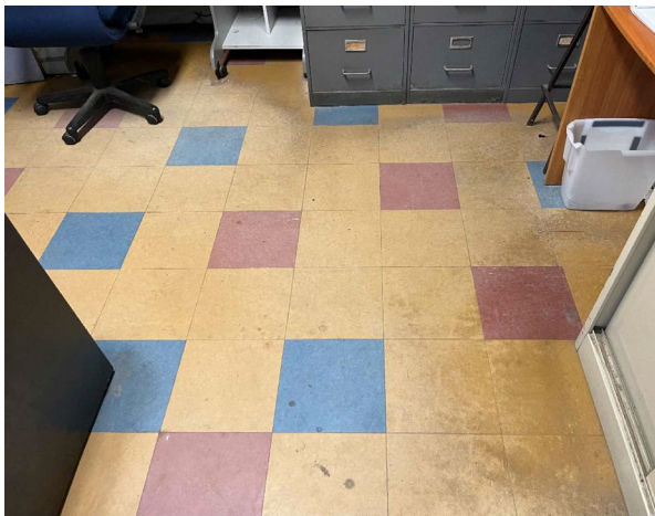
Line ID 37: Internal, GF, Maintenance Office, Floor Covering, Various Throughout, Vinyl Floor Tiles (blue) - Chrysotile Asbestos Detected
