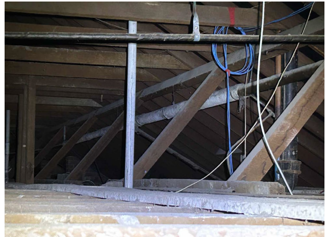
Line ID 92: Internal, L1, Southeast Wing, Ceiling Space, Central, Pipework, Lagging - Amosite Asbestos Detected
