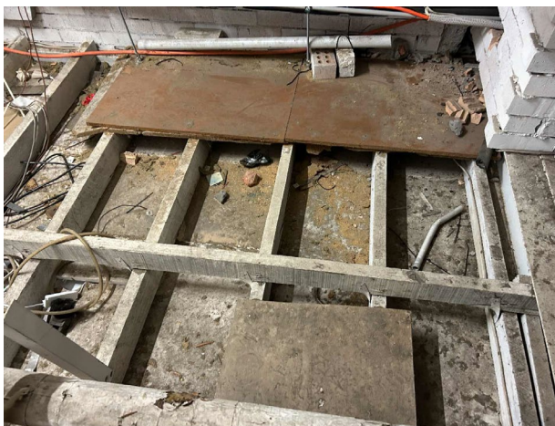
Line ID 126: Internal, GF, Central Wing, Ward A & B, Ceiling Space, All surfaces, Throughout, Dust - Lead Detected (900mg/kg)
