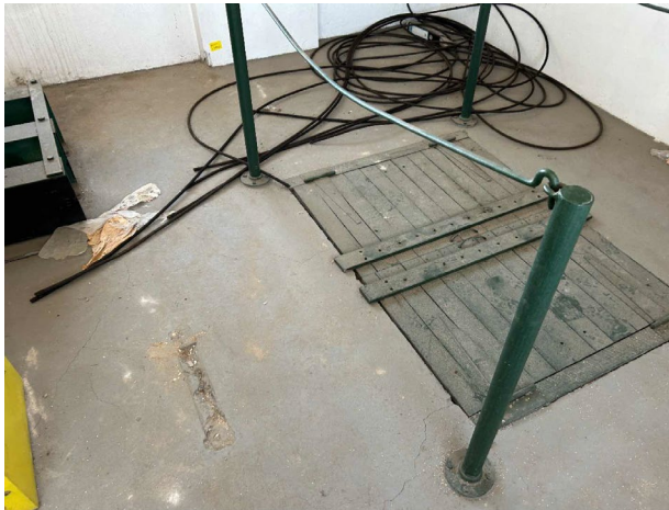
Line ID 130: Internal, L2, Lift Motor Room, On Floor, Dust - Lead Detected (3,300 mg/kg)
