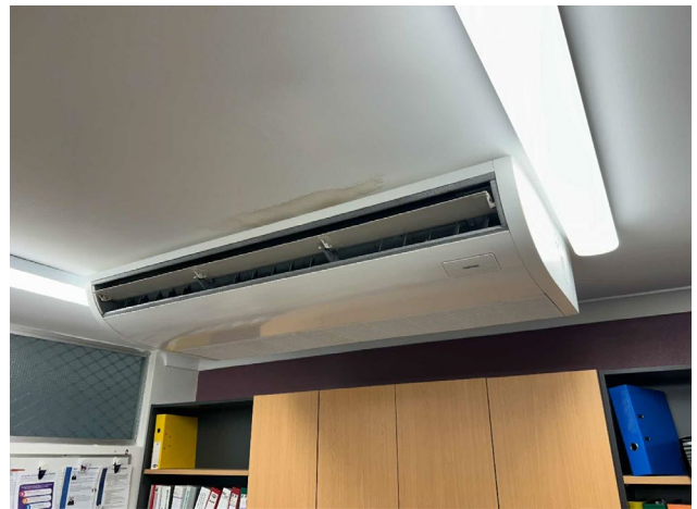
Line ID 171: Internal, GF, Central Wing, North Section, Pharmacy 1075, AC Unit, Unknown Refrigerant - Suspected ODS
