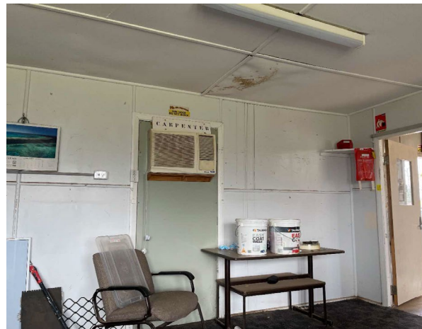
Line ID 44: Internal, GF, Workshops, Central Section, Wall & Ceiling Lining, Blue (Light) Paint - Lead Detected (0.25% w/w)
