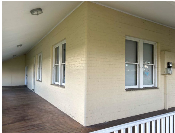
Line ID 27: External, GF, Cessnock House, East Wing, Walls, Cream Paint - Lead Detected (0.02% w/w)
