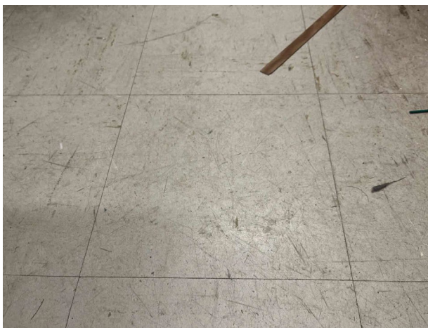
Line ID 73.1: Internal, GF, Central Wing, Ward B, Floor Covering, Room 1178, Throughout, Vinyl Floor Tiles (white) - Chrysotile Asbestos Detected
