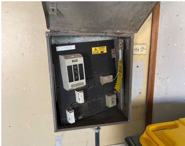
Line ID 23: Internal, GF, Workshops, Northern Section, Electrical Distribution Board 19 - Incinerator, Compressed Bituminous Panel - Suspected Asbestos
