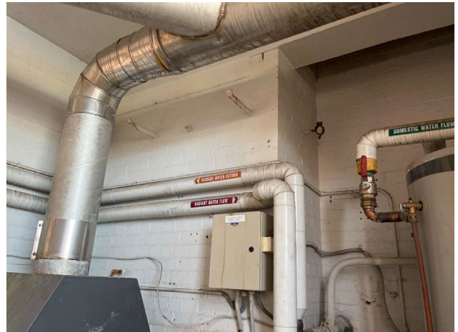
Line ID 140: Internal, GF, Central Wing, Day Surgery/Recovery, Plant Room, Pipework, Insulation Material - Suspected SMF
