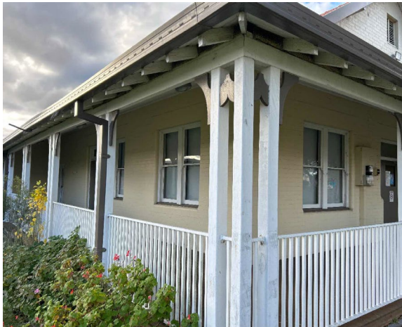
Line ID 26: External, GF, Cessnock House, East Wing, Veranda, Timberwork, White Paint - Lead Detected (2.6 % w/w)
