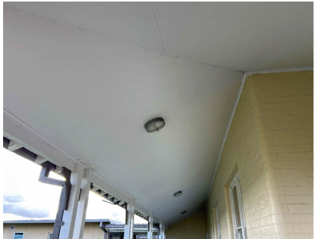
Line ID 2: External, GF, Cessnock House, East Wing, Veranda Ceiling, Fibre Cement Sheeting - No Asbestos Detected
