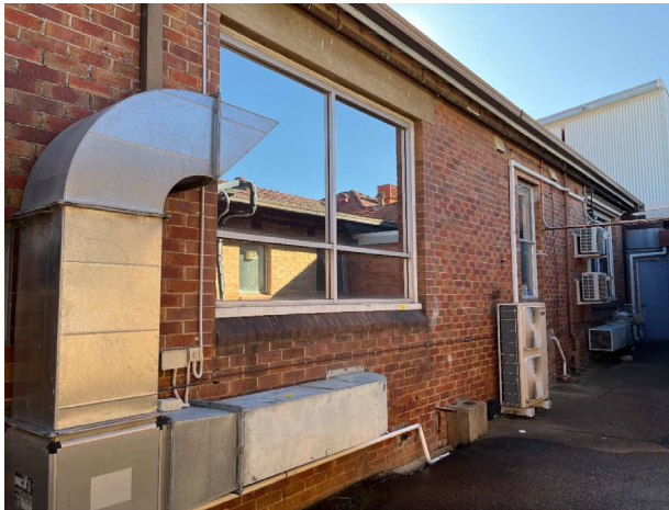
Line ID 108.1: External, GF, Central Wing, Northern Courtyard, Timber Window Frames, White Paint - Lead Detected (1.8% w/w)
