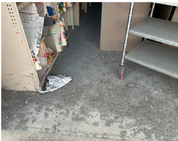
Line ID 50: Internal, GF, Workshops, Southern Section, Floor, Dust - Lead Detected (1,500 mg/kg)
