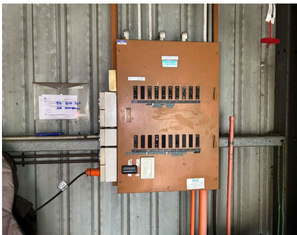
Line ID 14: Internal, GF, Northern Metal Shed, North, Distribution Board, Electrical Components - Suspected Asbestos
