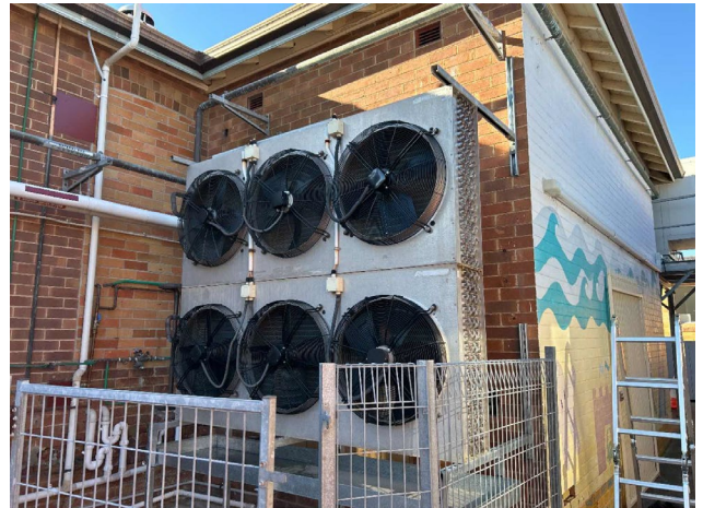
Line ID 164: External, GF, Central Wing, Northern Boiler Area, Chillers, Unknown Refrigerant - Suspected ODS
