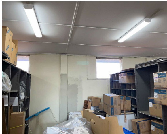
Line ID 13.1: Internal, GF, Storeroom, Wall Lining, Throughout, Cream Paint - Lead Detected (0.03% w/w)
