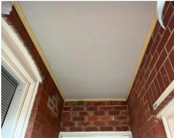
Line ID 1: External, GF, 1006 Entrance, Ceiling Lining, Throughout, Fibre Cement Sheet - No Asbestos Detected
