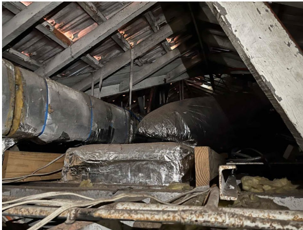
Line ID 147: Internal, GF, Central Wing, North Section, Plant Room 1119, Ceiling Space, Ductwork, Insulation Material - Suspected SMF
