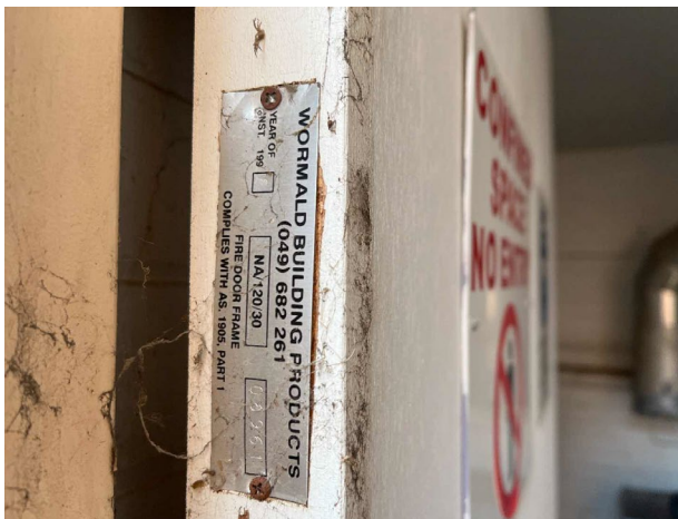
Line ID 13.1: External, GF, Central Wing, Southeast Side, Plant Room, Entrance Door, Fire Door Core - Suspected Asbestos
