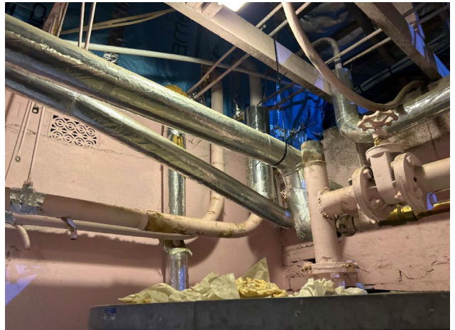
Line ID 146: Internal, GF, Central Wing, North Section, Plant Room 1073, Pipework Above Boilers, Insulation Material - Suspected SMF
