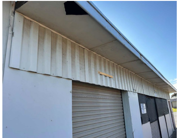
Line ID 13.1: External, GF, Workshops, All Areas, North and South Sections, Upper Walls, Profiled Cement Sheetting - Chrysotile Asbestos Detected
