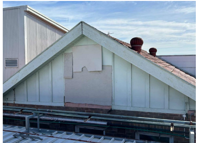
Line ID 29: External, Roof, Central Wing, North Section, Central Area, Infill Panels Below Roof Gable, Fibre Cement Sheeting - Chrysotile, Amosite and Crocidolite Asbestos Detected
