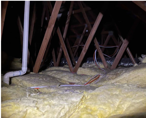
Line ID 36: Internal, GF, Cessnock House, West Wing - Ceiling Space, Flexible Ductwork, Insulation Material - Suspected SMF
