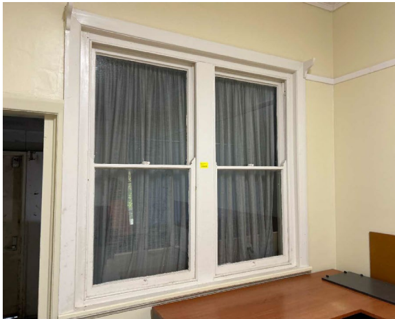
Line ID 30: Internal, GF, Cessnock House, East Wing, Window Frames, White Paint - Lead Detected (2.0% w/w)
