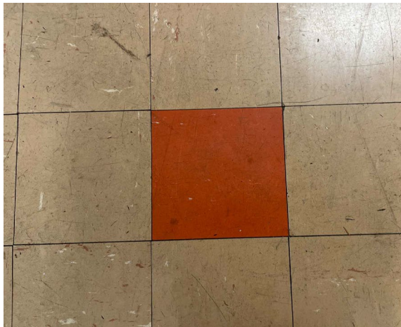
Line ID 7.1: Internal, GF, Storeroom, Main Foyer & Offices, Various Throughout, Vinyl Floor Tiles (red) - Chrysotile Asbestos Detected
