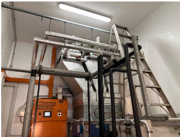
Line ID 149: Internal, GF, Central Wing, North Section, Plant Room 1119, Ductwork, Insulation Material - Suspected SMF
