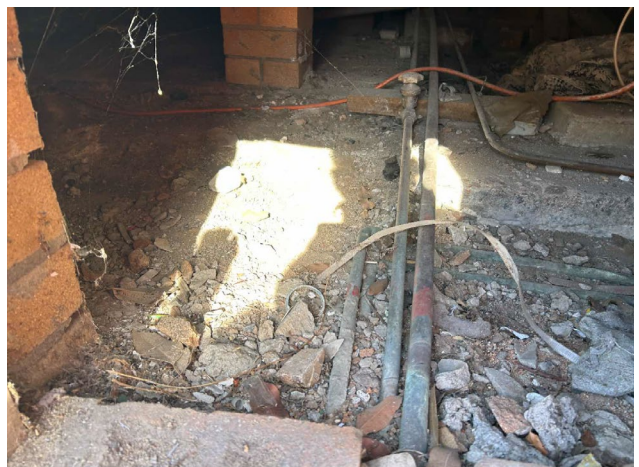
Line ID 64: Internal, GF, Central Wing, North Section, Sub-Floor Area, Central North, Adjacent Hatch, Fibre Cement Sheeting - Chrysotile Asbestos Detected
