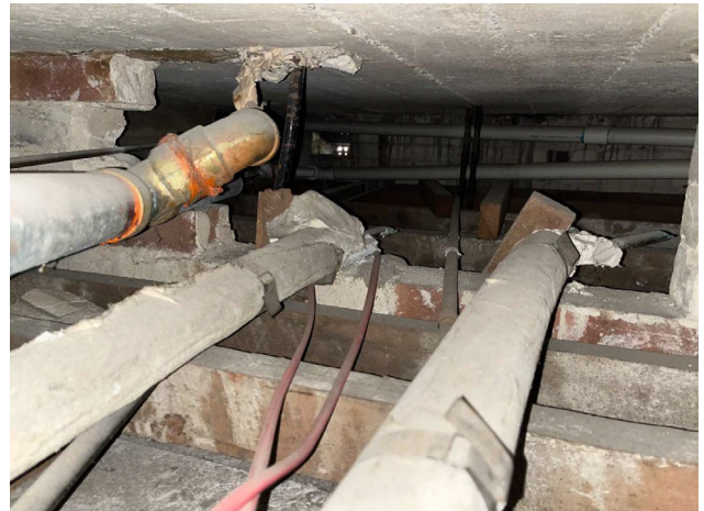
Line ID 80.1: Internal, GF, Southeast Wing, Ceiling Space, Throughout, Lagging - Amosite Asbestos Detected
