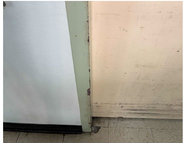
Line ID 20: Internal, GF, Kitchen, Door Frames, Throughout, Green (Light) Paint - Lead Detected (0.099% w/w)
