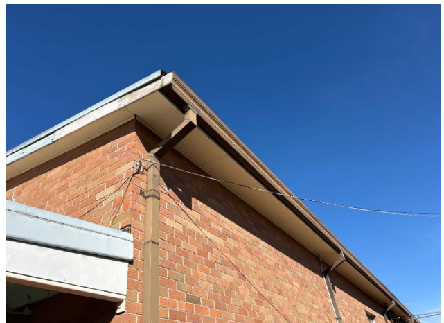
Line ID 3: External, GF, Central Wing, North Side, Eaves, Fibre Cement Sheeting - No Asbestos Detected
