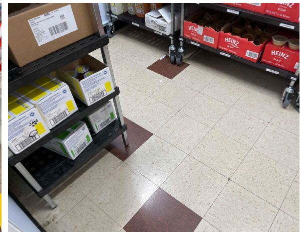
Line ID 13: Internal, GF, Kitchen, Room 1012, Throughout, Vinyl Floor Tiles (white with brown specs) - Chrysotile Asbestos Detected
