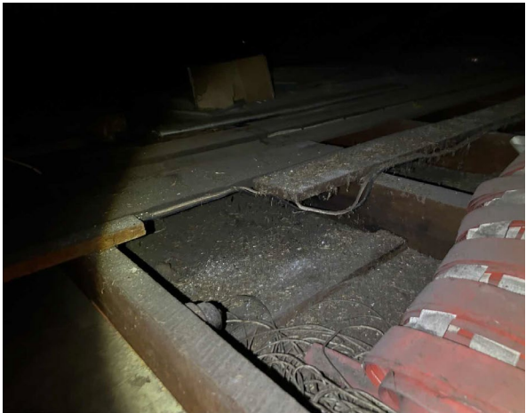
Line ID 49: Internal, GF, Workshops, Central Section, Throughout Ceiling Space, Dust - Lead Detected (5,400 mg/kg)
