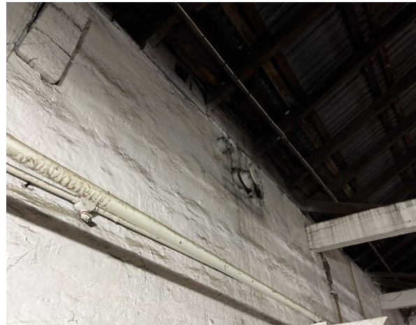
Line ID 39.1: Internal, GF, Painters Shop, Pipework Penetration, Northeast Adjacent Generator, Lagging - Amosite Asbestos Detected
