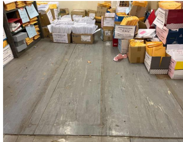
Line ID 16: Internal, GF, Document Storage Area, Floor covering, Adjacent entrance, Sheet Vinyl (grey) - No Asbestos Detected
