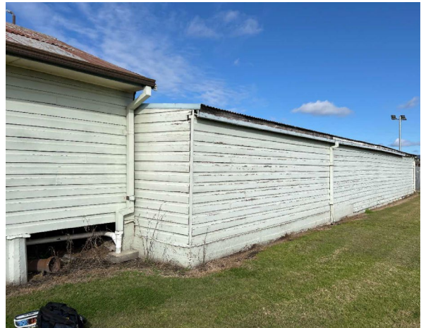
Line ID 36: External, GF, Workshops, All Areas, Central and South Sections, Timber Walls, White Paint - Lead Detected (0.18% w/w)
