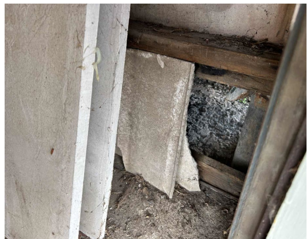
Line ID 28: Internal, GF, Workshops, Southern Section, Unit 1008, North, Lower Infill Panels, Profiled Cement Sheeting - Chrysotile Asbestos Detected
