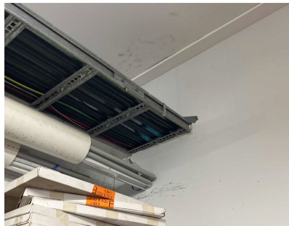
Line ID 65: Internal, GF, Main Workshop Area, Pillow Insulation, Cable Penetration, East, Insulation Material - Suspected SMF
