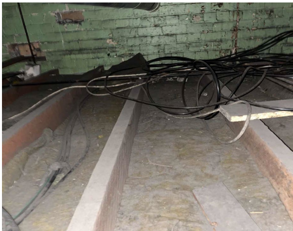
Line ID 57: Internal, GF, 1044, Painters Room, Ceiling Space, Insulation Batts - Suspected SMF
