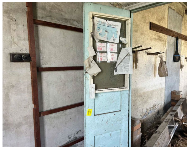
Line ID 40: Internal, GF, Old Mortuary, Central Door and Frame, Blue Paint - Lead Detected (12% w/w)
