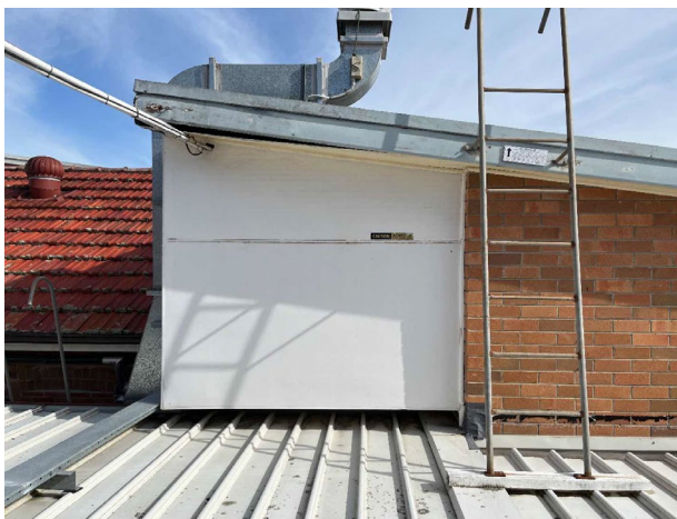
Line ID 30: External, Roof, Central Wing, North Section, Infill Panel, Adjacent Ladder Access, Fibre Cement Sheeting - No Asbestos Detected
