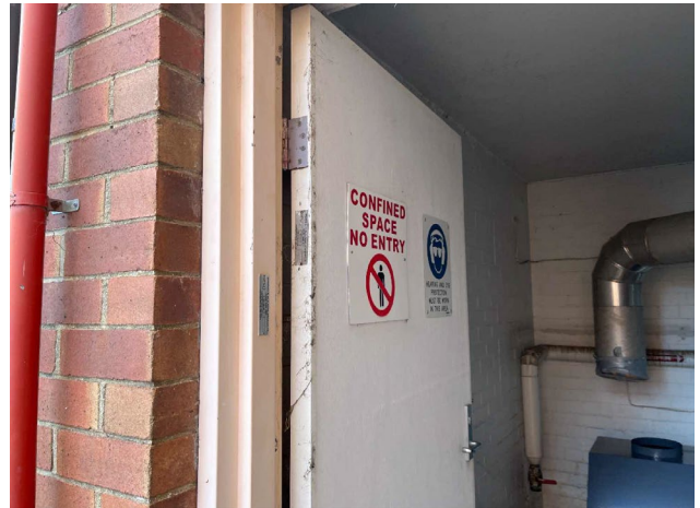
Line ID 13: External, GF, Central Wing, Southeast Side, Plant Room, Entrance Door, Fire Door Core - Suspected Asbestos
