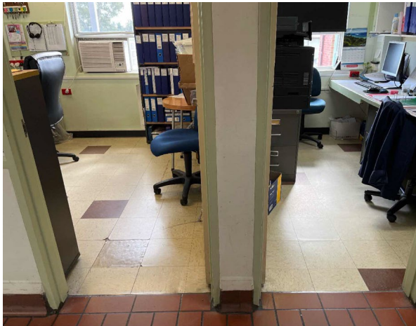
Line ID 14: Internal, GF, Kitchen, Rooms 1008 & 1007, Throughout, Vinyl Floor Tiles (white with brown specs) - Chrysotile Asbestos Detected
