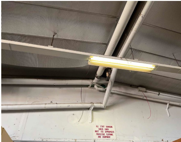
Line ID 25: Internal, GF, Laundry, Pipework, North East, Gasket Material - Chrysotile Asbestos Detected
