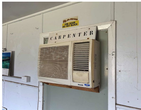
Line ID 57: Internal, GF, Workshops, Central Section, Central Office, AC Unit, R22 Hydrochlorofluorocarbon (HCFC) - ODS Refrigerant
