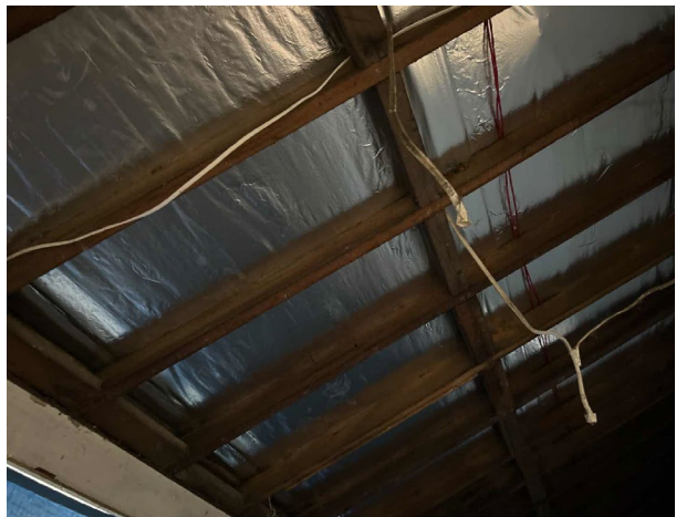
Line ID 35: Internal, GF, Cessnock House, East Wing, Northeast Covered Veranda Room, Ceiling, Sarking Insulation - Suspected SMF
