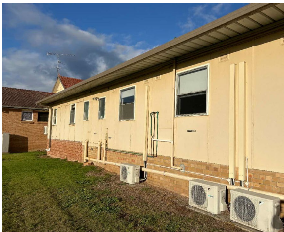
Line ID 28: External, GF, Pathology, South Wall, Cream Paint - Lead Detected (0.19% w/w)
