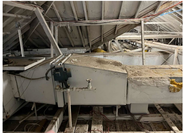
Line ID 152: Internal, GF, Central Wing, Ward A & B, Ceiling Space, Ductwork, Insulation Material - Suspected SMF
