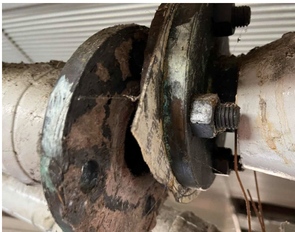
Line ID 24: Internal, GF, Laundry, Pipework, Central, Gasket Material - Chrysotile Asbestos Detected
