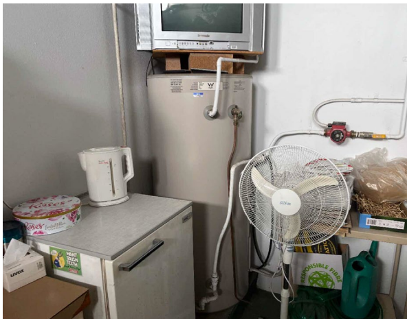
Line ID 61: Internal, GF, Kitchenette, Hot Water Heater, Adjacent Entry, Internal Insulation Material - Suspected SMF
