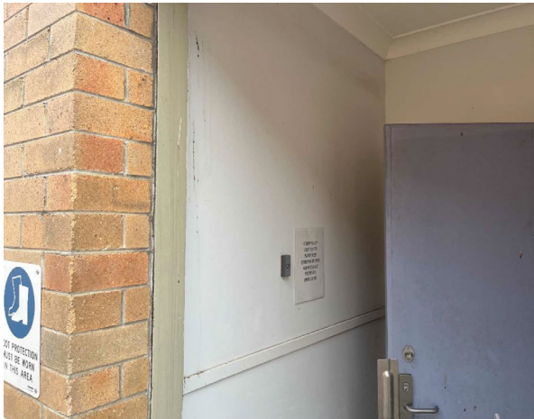
Line ID 33.1: Internal, GF, Main Workshop Area, Entrance Adjacent Toilet, Wall Lining, Fibre Cement Sheetting - No Asbestos Detected
