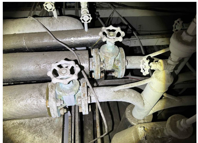
Line ID 38: Internal, GF, Central Wing, Day Surgery/Recovery, Ceiling Space Above Reception Area, Pipework, Gasket Material - Chrysotile Asbestos Detected
