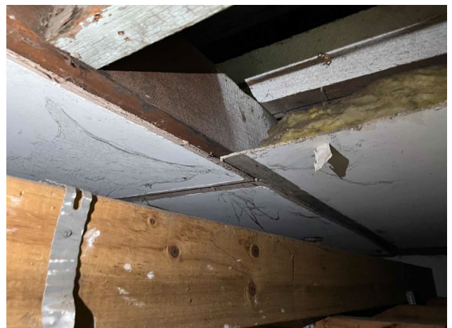
Line ID 58: Internal, GF, Central Wing, North Section, Plant Room 1119, Ceiling Space, Ceiling, Fibre Cement Sheeting - Chrysotile Asbestos Detected
