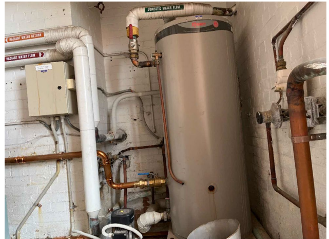
Line ID 142: Internal, GF, Central Wing, Day Surgery/Recovery, Plant Room, Water Heater, Insulation Material - Suspected SMF
