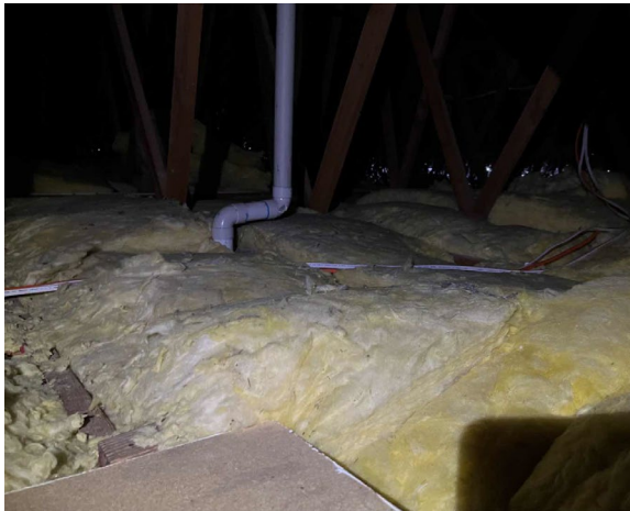
Line ID 38: Internal, GF, Cessnock House, West Wing - Ceiling Space, Throughout, Insulation Batt's - Suspected SMF
