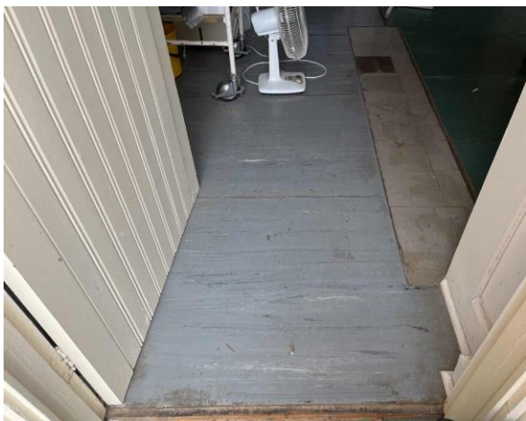
Line ID 12: Internal, GF, Dining/Laundry, Floor covering, Adjacent Entrance, Sheet Vinyl (grey) - No Asbestos Detected
