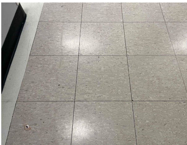
Line ID 78.1: Internal, GF, Central Wing, Ward B, Rooms 1174, 1176 & 1177, Floor Covering, Vinyl Floor Tiles (white with grey specks) - Chrysotile Asbestos Detected
