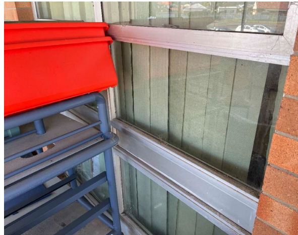
Line ID 6: External, GF, All Areas, Metal Windows, Throughout, Window Caulking - Chrysotile Asbestos Detected
