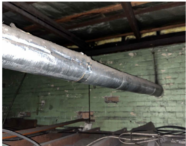
Line ID 58: Internal, GF, 1044, Painters Room, Ceiling Space, Pipework, Insulation Material - Suspected SMF
