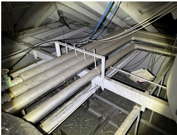
Line ID 136: Internal, GF, All Areas, Ceiling Space, Pipework, Insulation Material - Suspected SMF
