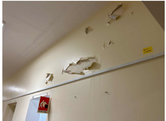
Line ID 119: Internal, L1, Southeast Wing, All Areas, Walls, Cream Paint - Lead Detected (0.30% w/w)
