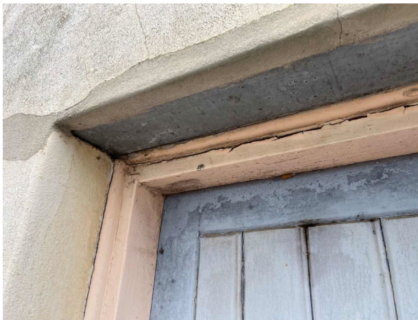
Line ID 109.1: External, GF, Southeast Wing, Door & Frames, Various Throughout, Pink (Light) Paint - Lead Detected (0.02% w/w)
