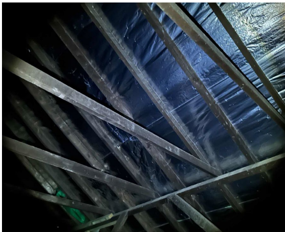
Line ID 34: Internal, GF, Cessnock House, East Wing, Ceiling Space, Sarking Insulation - Suspected SMF
