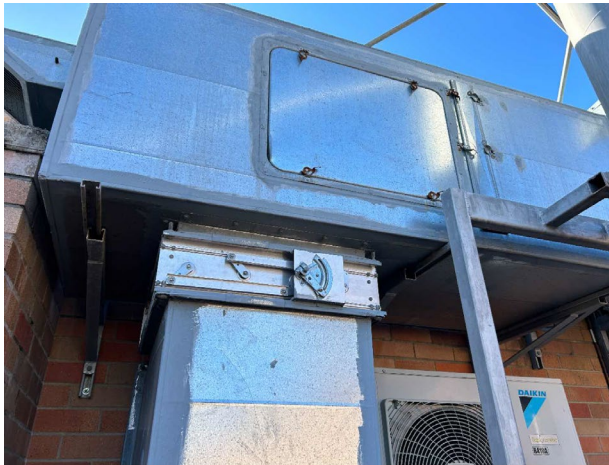
Line ID 6: External, GF, Central Wing, Northern Boiler Area, Ductwork Flange Joints, Mastic Sealant - No Asbestos Detected
