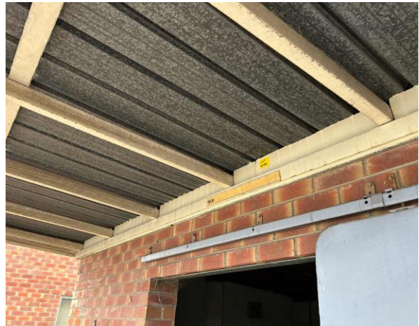
Line ID 5: External, GF, Dangerous Goods Store, West, Fascia, Fibre Cement Sheeting - Chrysotile, Amosite and Crocidolite Asbestos Detected
