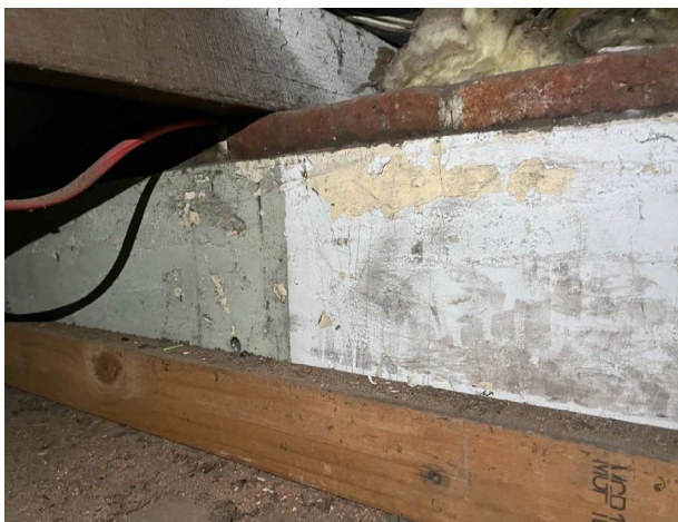
Line ID 115: Internal, GF, Central Wing, North Section, Plant Room 1119, Ceiling Space, Walls, White Paint - Lead Detected (0.02% w/w)
