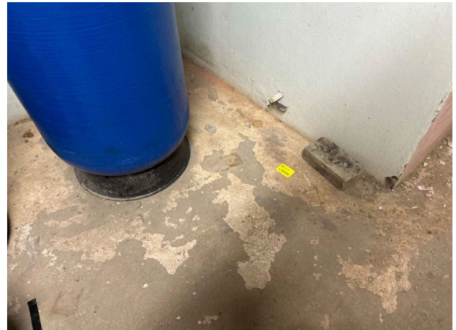
Line ID 114: Internal, GF, Central Wing, North Section, Plant Room 1073, Floor, Cream Paint - Lead Detected (0.03% w/w)
