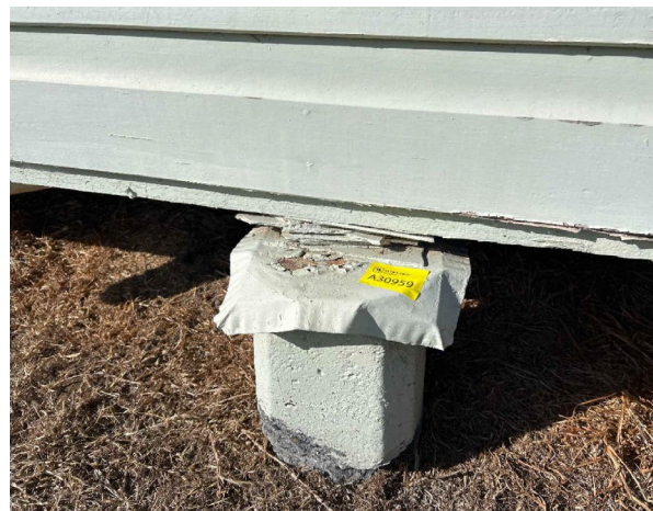
Line ID 7: External, GF, Workshops, All Areas, Central Section, Subfloor, Packing, Fibre Cement Sheetting - Chrysotile Asbestos Detected
