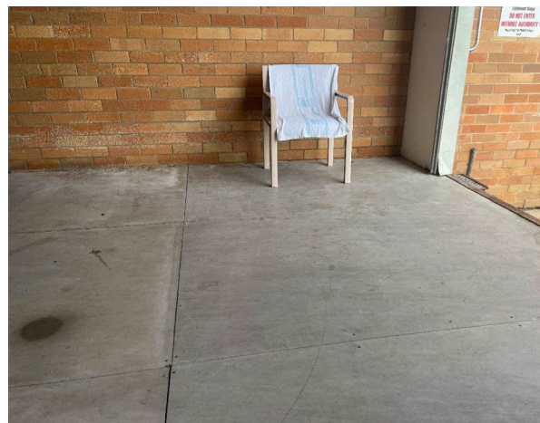
Line ID 42: Internal, GF, Palliative Care Storage Loading Dock, Floor Covering, Throughout, Compressed Cement Sheeting - No Asbestos Detected
