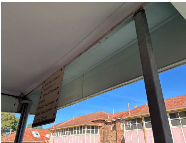
Line ID 25.1: External, GF, West Wing, Western Covered Area Adjacent Kitchen, Awning and Infill Panels, Fibre Cement Sheetting - Chrysotile Asbestos Detected
