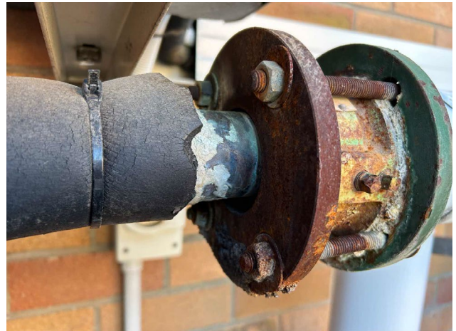
Line ID 9: External, GF, Central Wing, Northern Boiler Area, Residue to Pipework, Lagging - No Asbestos Detected
