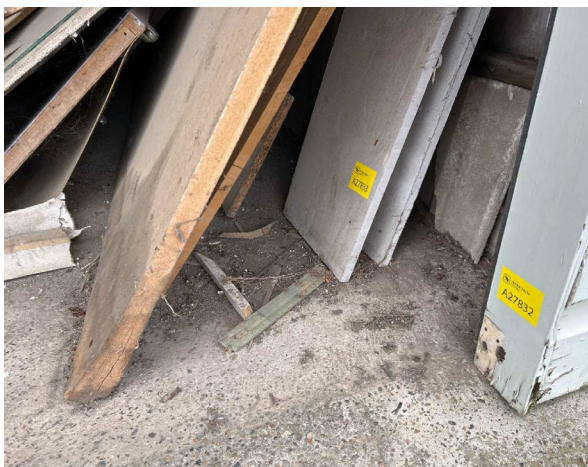
Line ID 27: Internal, GF, Workshops, Southern Section, Unit 1008, Floor, Dust - Chrysotile Asbestos Detected
