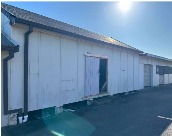
Line ID 5: External, GF, Workshops, All Areas, Central and North Sections, Walls, Fibre Cement Sheeting - Chrysotile, Amosite and Crocidolite Asbestos Detected
