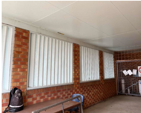
Line ID 11.1: External, GF, Mortuary, All Areas, Timber Works, Adjacent Entrance, Blue (Light) Paint - Lead Detected (0.23% w/w)
