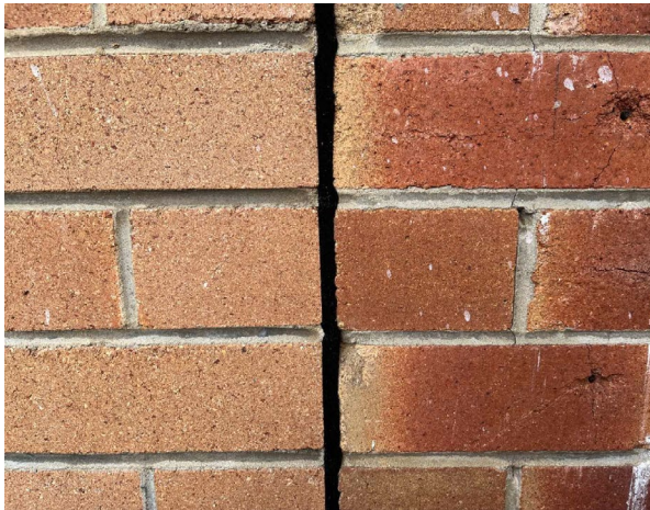
Line ID 6.1: External, GF, All Areas, Southwest, Between Brick, Adjacent Doctor Parking Spot, Construction Joint Mastic - No Asbestos Detected
