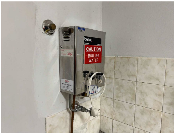
Line ID 159: Internal, GF, Southeast Wing, Room 1191, Water Heater, Insulation Material - Suspected SMF
