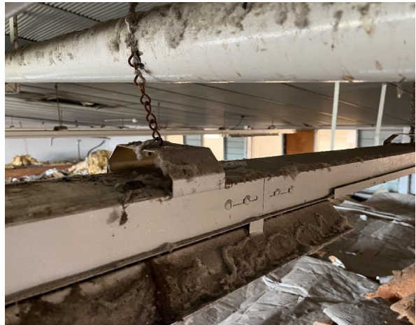
Line ID 22: Internal, GF, Laundry, High Level Surfaces, Throughout, Dust - No Asbestos Detected
