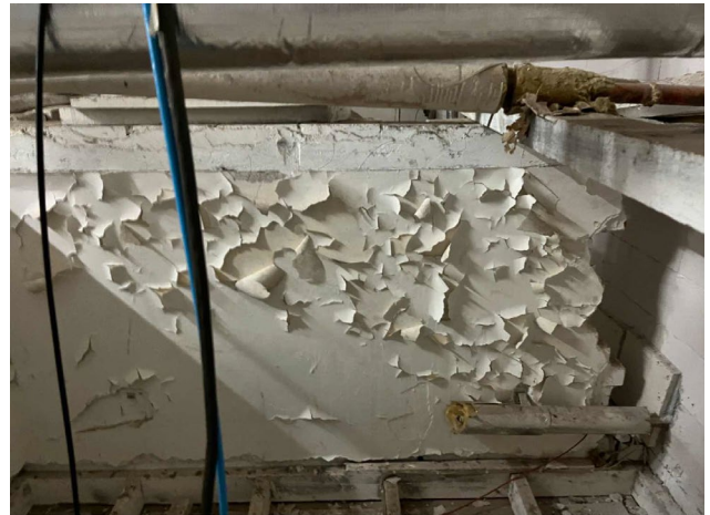
Line ID 117.1: Internal, GF, Central Wing, Ward A & B, Ceiling Space, Brickwork Lining, White Paint - Lead Detected (4.1% w/w)
