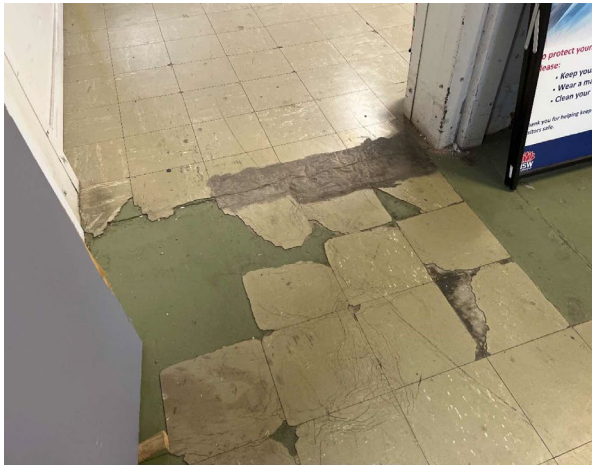
Line ID 19: Internal, GF, Laundry, Floor Covering, Throughout, Vinyl Floor Tiles (grey with white specs, large squares) - Chrysotile Asbestos Detected
