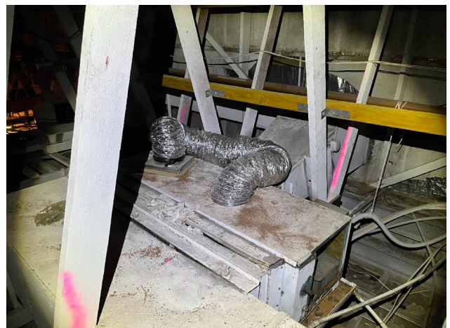
Line ID 144: Internal, GF, Central Wing, North Section, Ceiling Space, Flexible Ductwork, Throughout, Insulation Material - Suspected SMF
