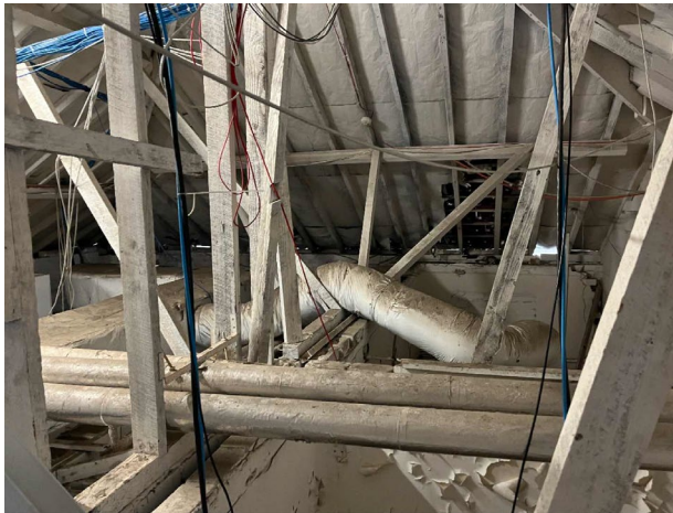
Line ID 153: Internal, GF, Central Wing, Ward A & B, Ceiling Space, Flexible ductwork, Insulation Material - Suspected SMF
