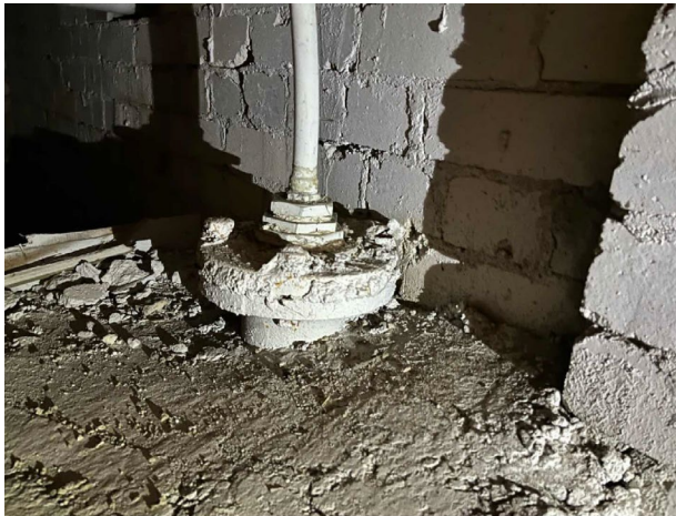
Line ID 89: Internal, GF, Southeast Wing, Southern Sub-Floor Area, Central, Pipework, Gasket Material - No Asbestos Detected
