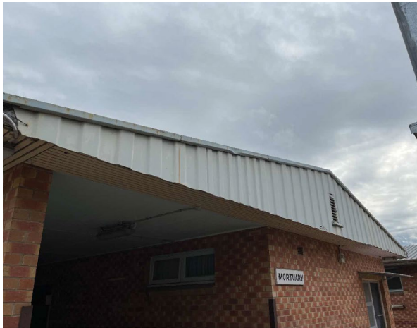
Line ID 2: External, GF, Mortuary, All Areas, Gable End, North & South, Moulded Fibre Cement - Chrysotile and Amosite Asbestos Detected
