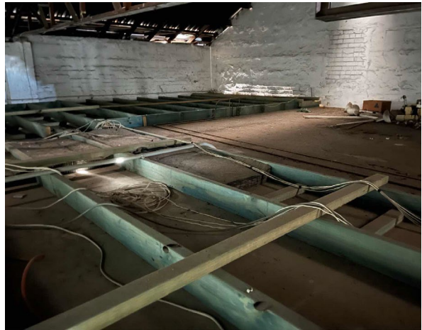
Line ID 55: Internal, GF, Painters Shop, Ceiling Space, Throughout, Dust - Lead Detected (220mg/kg)
