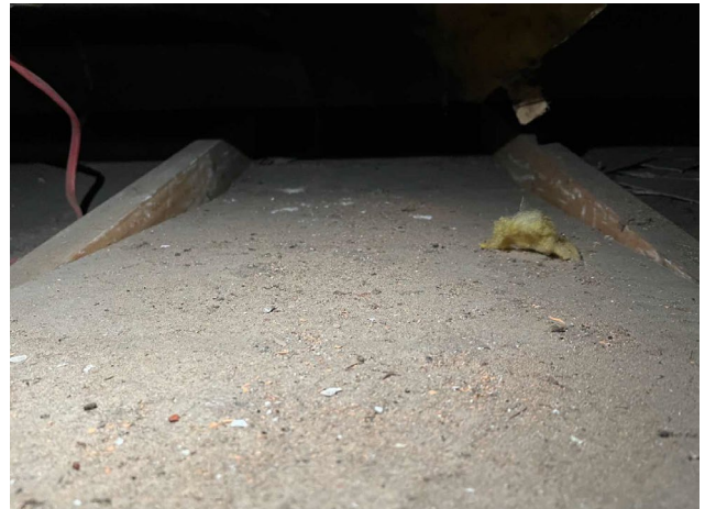
Line ID 125: Internal, GF, Central Wing, North Section, Plant Room 1119, Ceiling Space, Dust - Lead Detected (340mg/kg)
