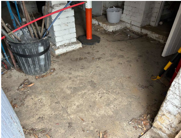
Line ID 128: Internal, GF, Southeast Wing, Southern Sub-Floor Area, Throughout, Dust - Lead Detected (740mg/kg)
