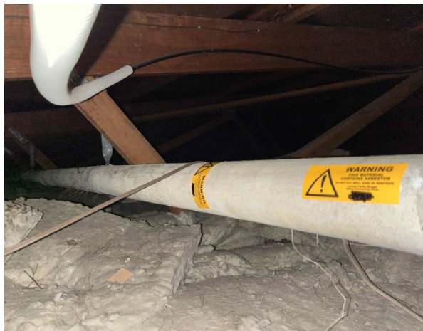
Line ID 9: Internal, GF, Storeroom Ceiling Space, Pipework, Throughout, Lagging - Amosite Asbestos Detected
