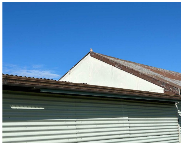
Line ID 4: External, GF, Workshops, All Areas, Central and North Sections, Roof Gable Panels, Fibre Cement Sheeting - Chrysotile, Amosite and Crocidolite Asbestos Detected
