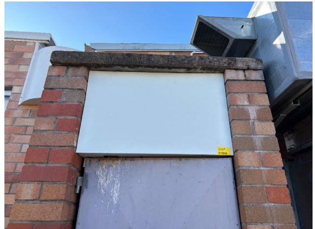
Line ID 7: External, GF, Central Wing, Northern Boiler Area, Infill Panel Above Oxygen Storage, Fibre Cement Sheetting - No Asbestos Detected
