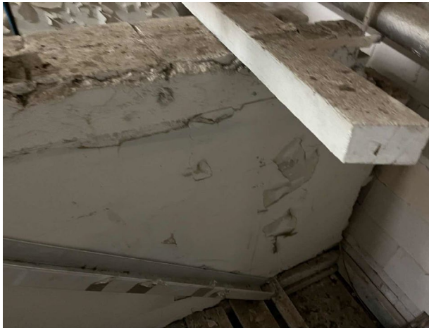
Line ID 117: Internal, GF, Central Wing, Ward A & B, Ceiling Space, Brickwork Lining, White Paint - Lead Detected (4.1% w/w)
