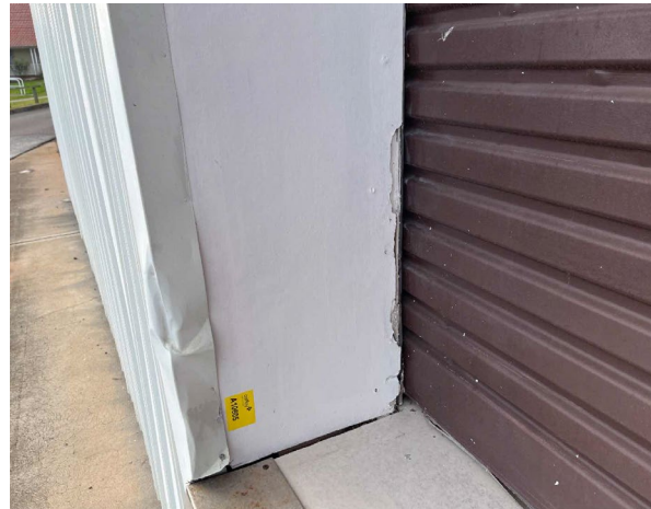
Line ID 9: External, GF, Palliative Care Equipment Room, Wall Lining, Roller door, Fibre Cement Sheeting - No Asbestos Detected
