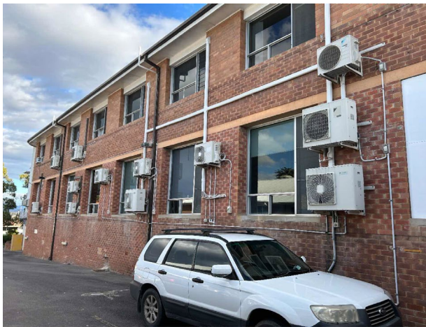
Line ID 170: External, GF and L1, Southeast Wing, East and West Sides, AC Units, R410A and R32 Hydrofluorocarbon (HFC) - Non ODS Refrigerant
