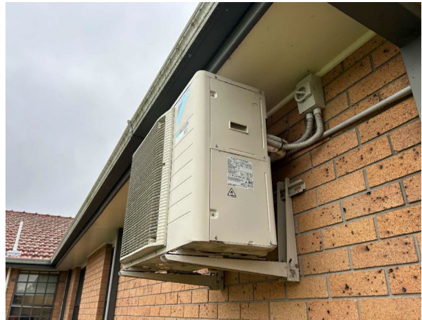
Line ID 43: External, GF, Cessnock House, West Wing, North, AC Units, R32 Refrigerant - Non ODS Refrigerant
