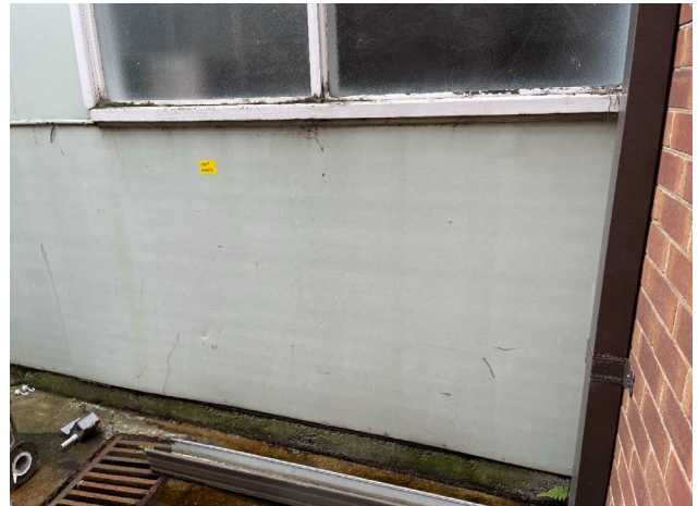
Line ID 2: External, GF, Central Wing, Central Courtyard, Wall Lining, Entry, Fibre Cement Sheeting - Chrysotile, Amosite and Crocidolite Asbestos Detected
