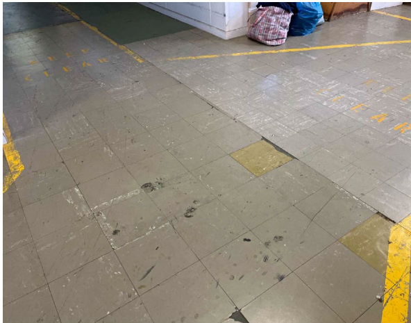
Line ID 21.1: Internal, GF, Laundry, Floor Covering, Various Throughout, Vinyl Floor Tiles (khaki green with white specs) - Chrysotile Asbestos Detected
