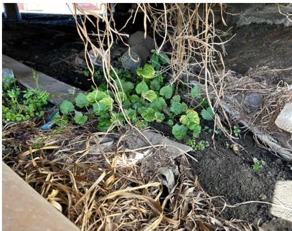
Line ID 6: External, GF, Workshops, All Areas, Central Section, Subfloor, Debris, Fibre Cement Debris - Chrysotile, Amosite and Crocidolite Asbestos Detected
