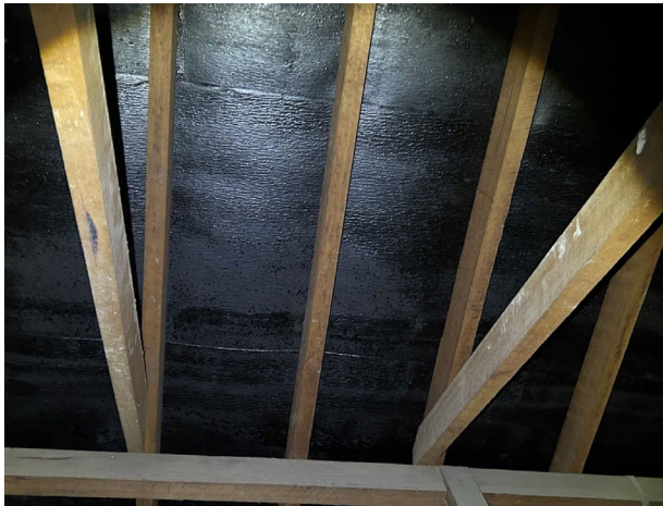
Line ID 95: Internal, L1, Southeast Wing, Ceiling Space, Waterproofing to Underside of Roof, Bituminous Material - Suspected Asbestos
