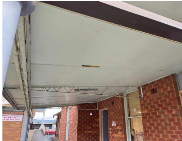
Line ID 7: External, GF, Front Entrance, Verandah, Awning, Fibre Cement Sheet - Chrysotile, Amosite and Crocidolite Asbestos Detected
