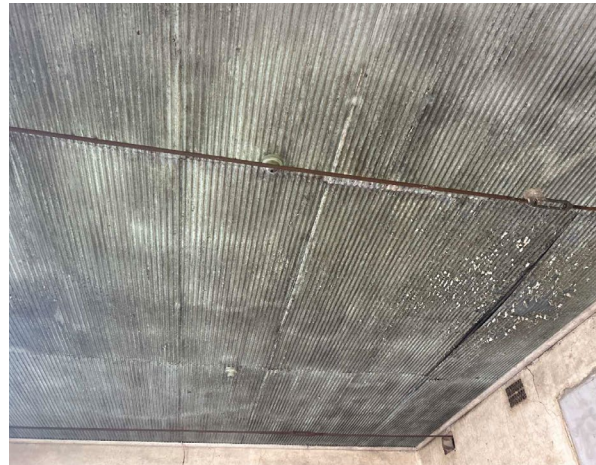
Line ID 42: Internal, GF, Old Mortuary, Throughout, Ceiling, Blue Paint - Lead Detected (12% w/w)
