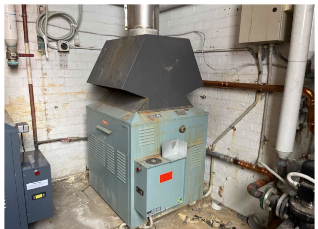
Line ID 139: Internal, GF, Central Wing, Day Surgery/Recovery, Plant Room, Boilers, Insulation Material - Suspected SMF
