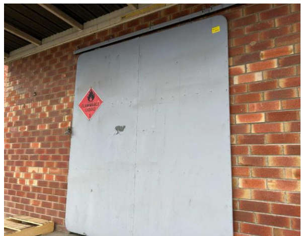
Line ID 22: External, GF, Dangerous Goods Store, Sliding Door, Purple Paint - Lead Detected (3.4% w/w)
