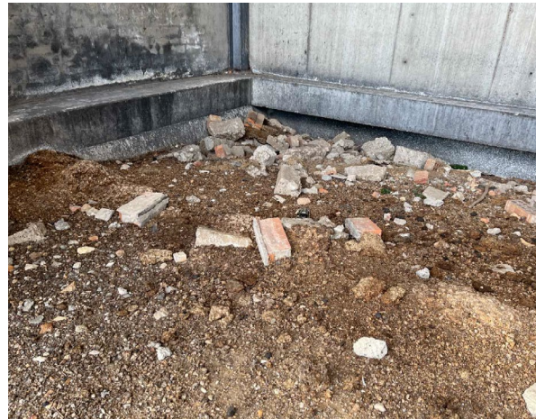
Line ID 10: External, GF, Room 1040, Old Coal Bunker, Floor, Throughout, Fibre Cement Debris - Chrysotile, Amosite and Crocidolite Asbestos Detected
