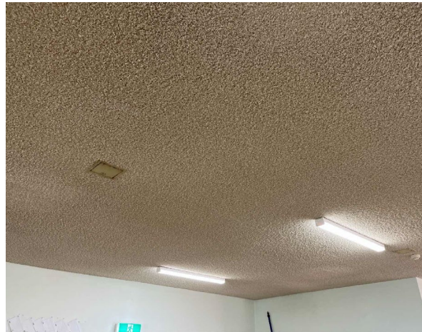
Line ID 8: Internal, GF, Kitchen Ceiling Lining, Throughout, Vermiculite - No Asbestos Detected
