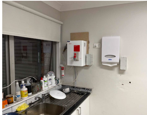
Line ID 60: Internal, GF, Kitchen, Hot Water Heater, Above Sink, Internal Insulation Material - Suspected SMF
