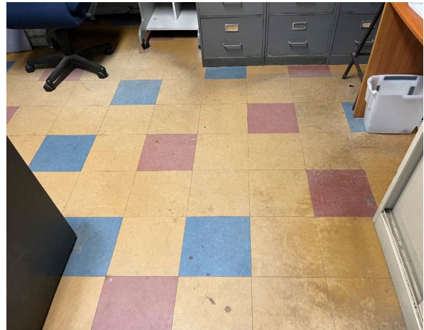
Line ID 36: Internal, GF, Maintenance Office, Floor Covering, Various Throughout, Vinyl Floor Tiles (red) - Chrysotile Asbestos Detected
