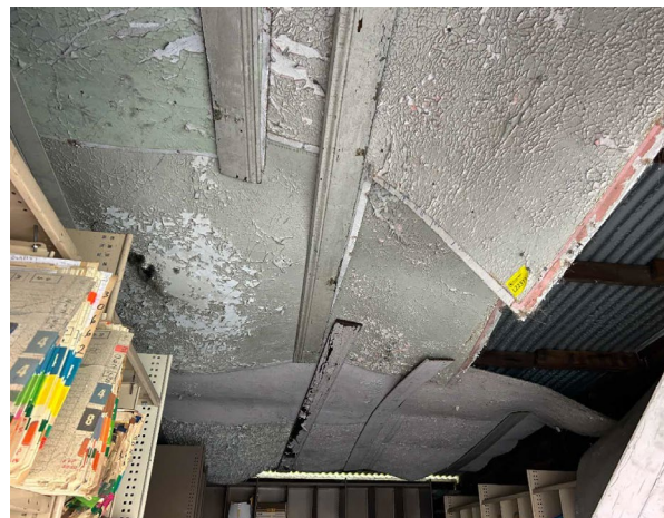
Line ID 45: Internal, GF, Workshops, Southern Section, Unit 1011, Ceiling, White Paint - Lead Detected (3.1% w/w)
