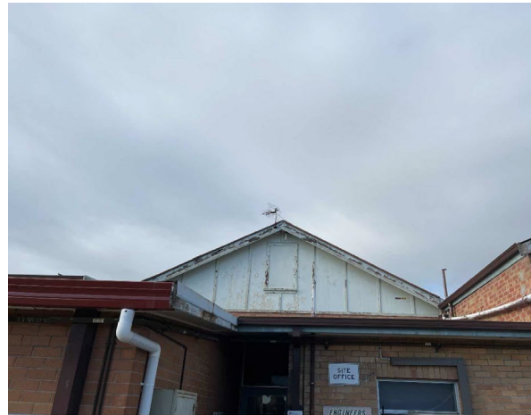
Line ID 3: External, GF, Gable End, Site Office Entrance, Roof, Fibre Cement Sheetting - Chrysotile Asbestos Detected
