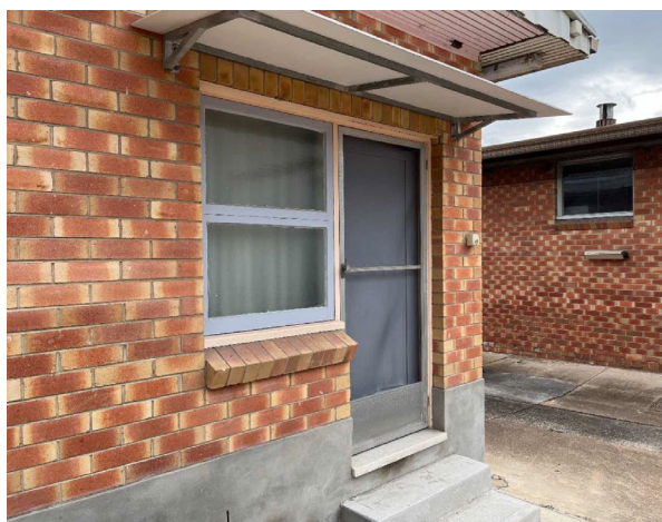
Line ID 10: External, GF, Mortuary, All Areas, Door & Frames, Throughout, Pink (Light) Paint - Lead Detected (0.18% w/w)
