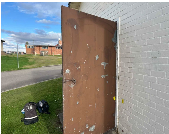
Line ID 33: External, GF, Old Mortuary, Entrance Door, Brown Paint - Lead Detected (0.096% w/w)
