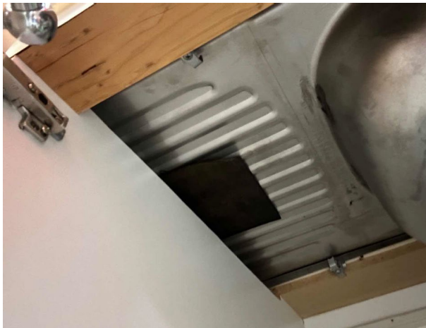
Line ID 49: Internal, GF, Central Wing, North Section, Pharmacy 1075, Sink Pad, Bituminous Material - Chrysotile Asbestos Detected
