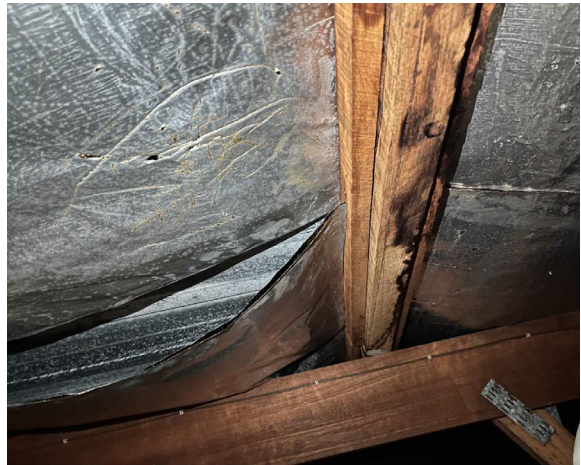
Line ID 16: Internal, GF, Storeroom Ceiling Space, Roof Lining, Sarking Insulation - Suspected SMF
