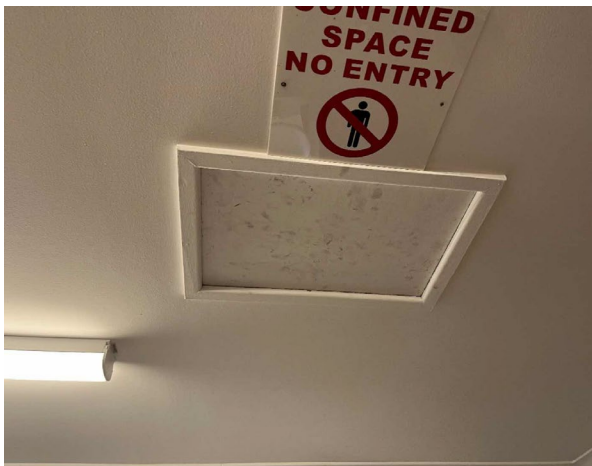
Line ID 13: Internal, GF, 1044, Painters Room, Access Hatch, Central, Fibre Cement Sheeting - No Asbestos Detected
