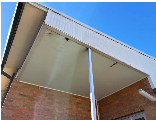
Line ID 4: External, GF, Central Wing, North Side, Entrance Awning Adjacent Room 1048, Fibre Cement Sheeting - No Asbestos Detected
