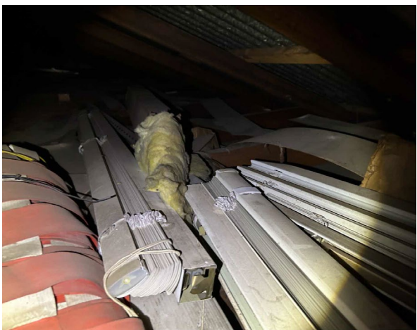
Line ID 51: Internal, GF, Workshops, Central Section, Ceiling Space, Insulation Batts - Suspected SMF
