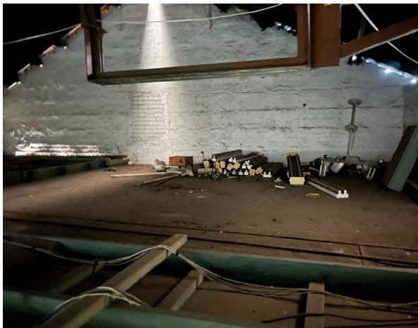
Line ID 70: Internal, GF, Painters Shop, Ceiling Space, Stored Item, Fluorescent Light Fitting, Capacitor(s) - Suspected PCB
