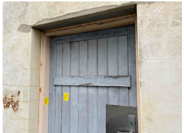
Line ID 110: External, GF, Southeast Wing, Door & Frames, Various Throughout, Purple (Light) Paint - Lead Detected (0.15% w/w)
