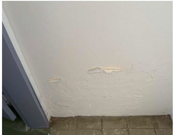
Line ID 53.1: Internal, GF, Room 1032, Toilet, Wall lining, Throughout, White Paint - Lead Detected (<0.005% w/w)
