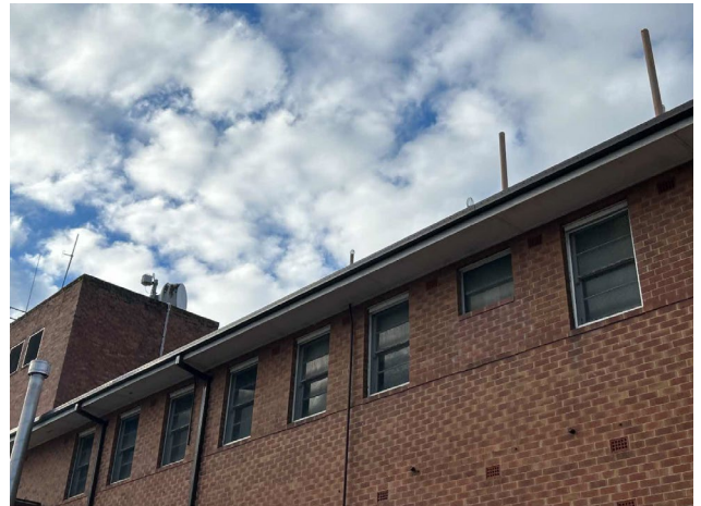
Line ID 27.1: External, L1, Southeast Wing, Throughout, Eaves, Fibre Cement Sheeting - Chrysotile Asbestos Detected
