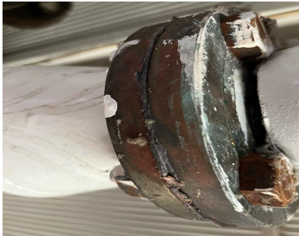
Line ID 23: Internal, GF, Laundry, Pipework, Central, Gasket Material - Chrysotile Asbestos Detected
