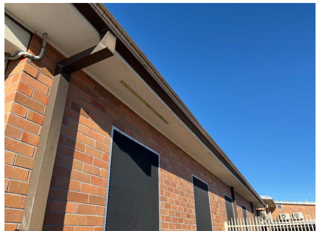
Line ID 14: External, GF, ED Wing, Eaves, Throughout, Fibre Cement Sheeting - Chrysotile Asbestos Detected
