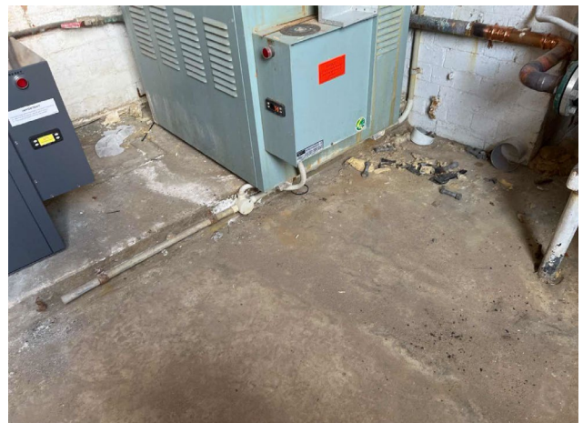
Line ID 121: Internal, GF, Central Wing, Day Surgery/Recovery, Plant Room, Throughout, Dust - Lead Detected (970mg/kg)
