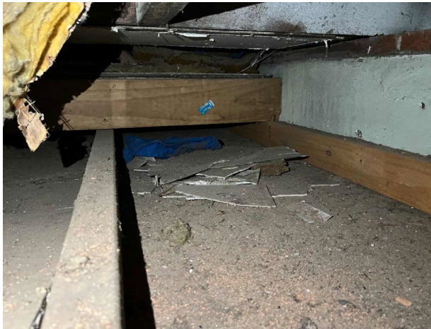
Line ID 59: Internal, GF, Central Wing, North Section, Plant Room 1119, Ceiling Space, Debris, Fibre Cement Debris - Chrysotile Asbestos Detected
