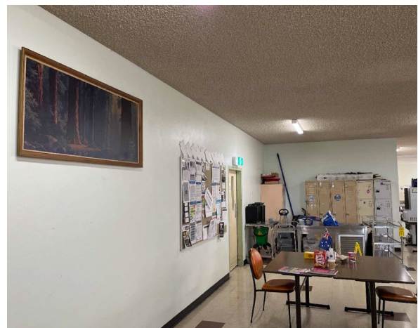
Line ID 21: Internal, GF, Kitchen, Wall lining, Throughout, Blue (Light) Paint - Lead Detected (0.02% w/w)
