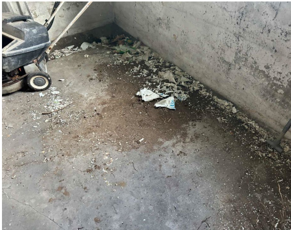
Line ID 41: Internal, GF, Old Mortuary, Debris on Floor, Cream Paint - Lead Detected (0.86% w/w)
