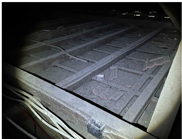
Line ID 12: Internal, GF, Cessnock House, East Wing, Ceiling Space, Dust - No Asbestos Detected
