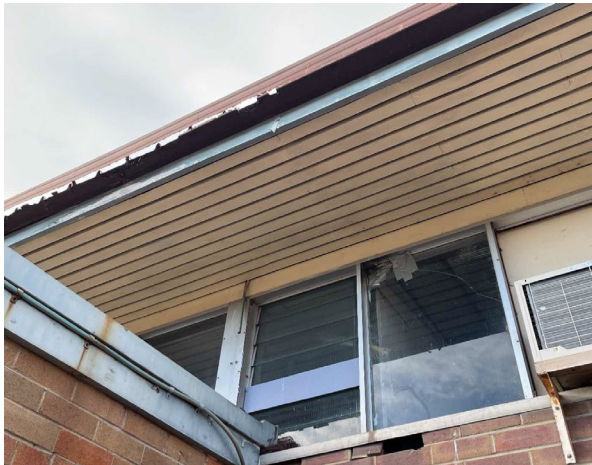
Line ID 5: External, GF, Infill Panel, Adjacent Site Office Roller Door, Above Window, Fibre Cement Sheeting - Chrysotile Asbestos Detected
