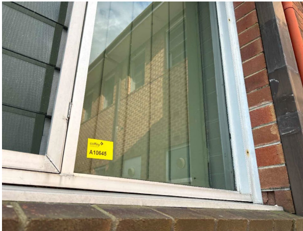
Line ID 12: External, GF, Central Wing, South Side, Metal Window Frames, Window Caulking - Chrysotile Asbestos Detected
