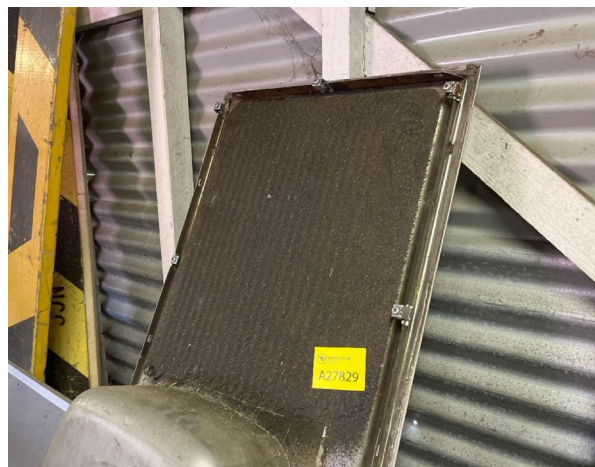
Line ID 24: Internal, GF, Workshops, Northern Section, Room 1004, Sink Pad, Bituminous Material - Chrysotile Asbestos Detected
