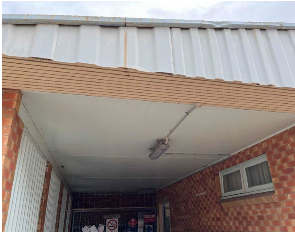
Line ID 1: External, GF, Mortuary, All Areas, Awning, Entrance, Fibre Cement Sheeting - Chrysotile Asbestos Detected
