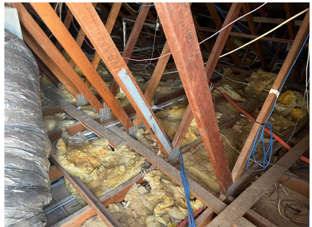
Line ID 156: Internal, GF, ED Wing, Ceiling Space, Insulation Batts, Throughout, Insulation Material - Suspected SMF
