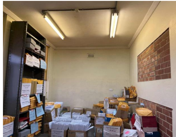
Line ID 24: Internal, GF, Document Storage Area, Wall lining, Throughout, Cream Paint - Lead Detected (0.24% w/w)
