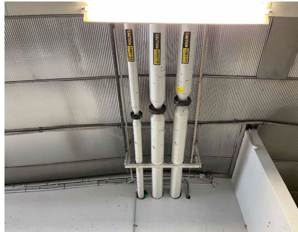
Line ID 26: Internal, GF, Laundry, Pipework, Southwest, Gasket Material - Chrysotile Asbestos Detected
