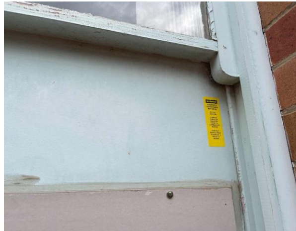
Line ID 2: External, GF, All Areas, Infill Panels, Below Windows, Fibre Cement Sheet - Chrysotile, Amosite and Crocidolite Asbestos Detected
