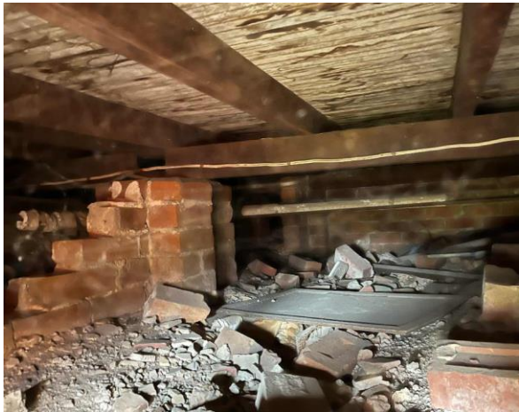
Line ID 9.1: External, GF, Subfloor Entrance, Pipework Lagging, Throughout, Lagging - Amosite Asbestos Detected
