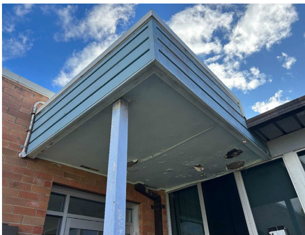
Line ID 21: External, GF, West Wing, Eastern Entrance Awning, Adjacent Room 1171, Fibre Cement Sheeting - Chrysotile & Amosite Asbestos Detected
