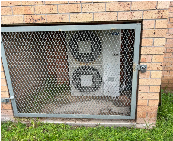
Line ID 42: External, GF, Cessnock House, West Wing, North Side, Below Stairs, AC Units, R22 Hydrochlorofluorocarbon (HCFC) - ODS Refrigerant
