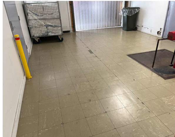
Line ID 19.1: Internal, GF, Laundry, Floor Covering, Throughout, Vinyl Floor Tiles (grey with white specs, large squares) - Chrysotile Asbestos Detected
