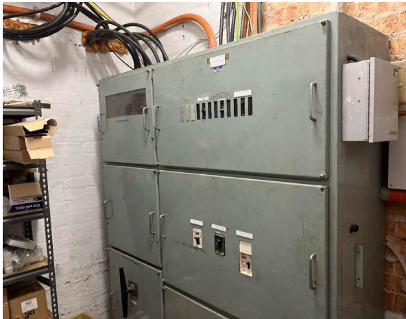
Line ID 29: Internal, GF, Main Switchboard Room, Electrical Distribution Board 1, Internal Electrical Components - Suspected Asbestos
