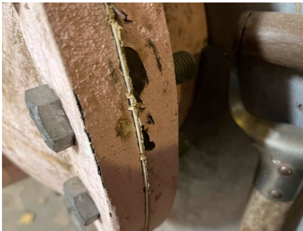
Line ID 51: Internal, GF, Central Wing, North Section, Plant Room 1073, Boiler, Large Gasket, Gasket Material - Chrysotile Asbestos Detected
