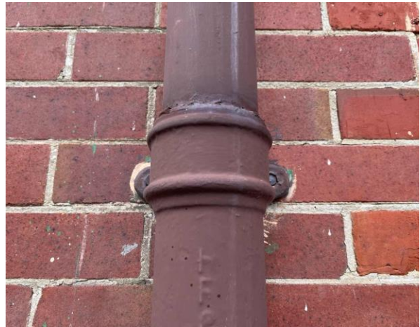
Line ID 20: External, GF, All Areas, Roof & Metal Work, Throughout, Brown Paint - Lead Detected (0.29% w/w)
