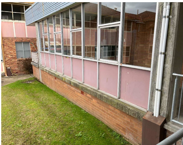
Line ID 4: External, GF, All Areas, Infill Panels, Below Windows, Fibre Cement Sheet - Chrysotile Asbestos Detected
