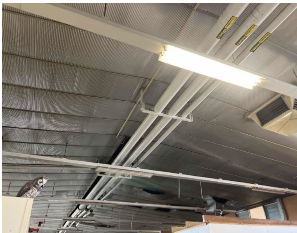
Line ID 27.1: Internal, GF, Laundry, Pipework, Throughout, Lagging - Amosite Asbestos Detected
