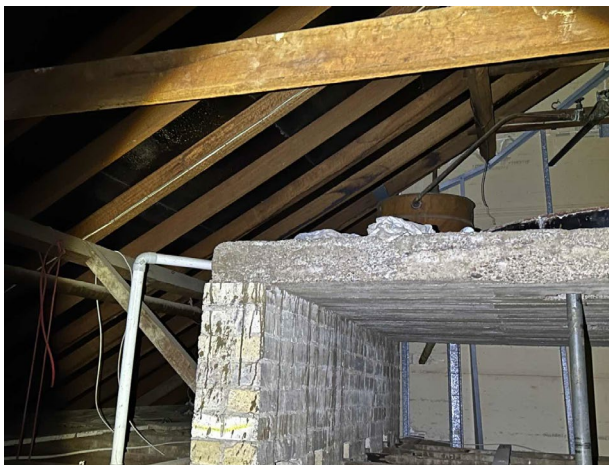
Line ID 93: Internal, L1, Southeast Wing, Ceiling Space, North, Stored On Ledge, Woven Material - Suspected Asbestos
