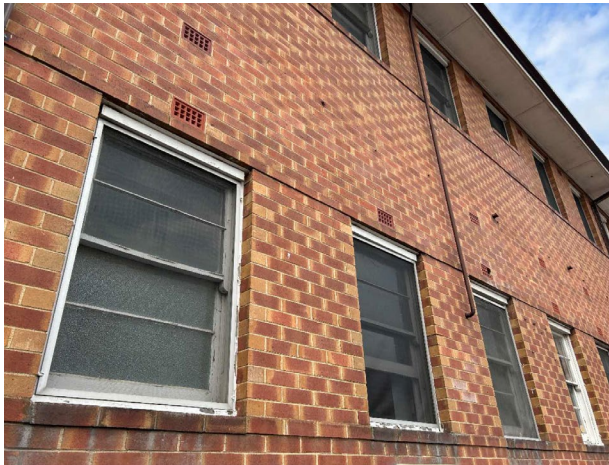
Line ID 111: External, GF and L1, Southeast Wing, Throughout, Timber Window Frames, White Paint - Lead Detected (4.7% w/w)
