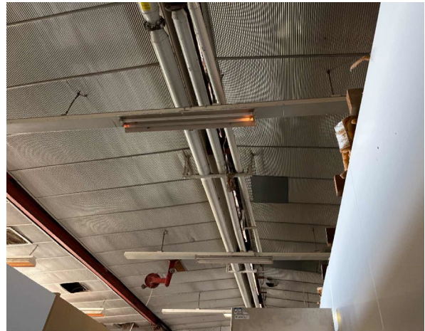
Line ID 69: Internal, GF, Laundry, Fluorescent Light Fitting, Throughout, Capacitor(s) - Suspected PCB
