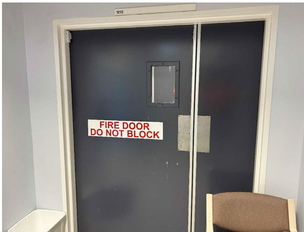
Line ID 81: Internal, GF, Southeast Wing, Double Door to Room 1213, Fire Door Core - Suspected Asbestos
