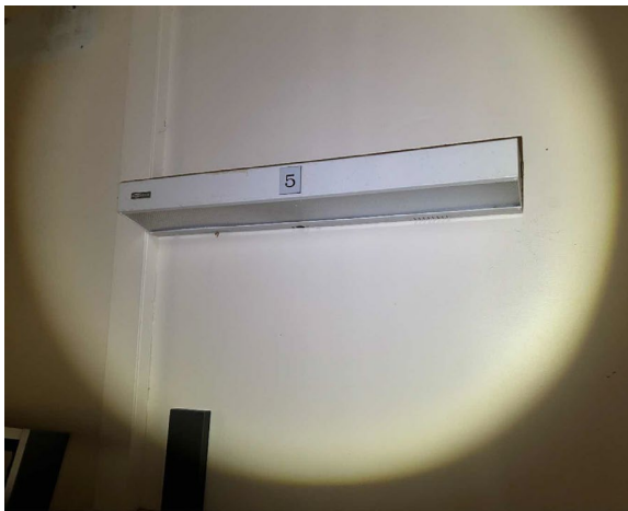
Line ID 40: Internal, GF, Cessnock House, East Wing, Original Wall Light Fittings, Capacitor(s) - Suspected PCB
