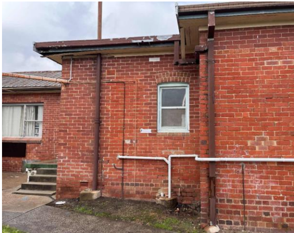
Line ID 20.1: External, GF, All Areas, Roof & Metal Work, Throughout, Brown Paint - Lead Detected (0.29% w/w)
