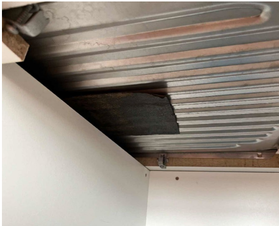
Line ID 20: Internal, GF, Pathology, Staff Room, Sink Pad, Bituminous Material - Chrysotile Asbestos Detected
