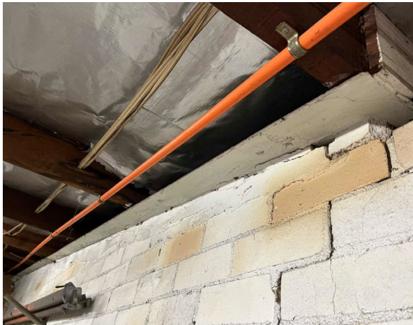
Line ID 47: Internal, GF, Room 1034, Storage, Packer/Ceiling Lining, South West, Fibre Cement Sheetting - Chrysotile and Amosite Asbestos Detected
