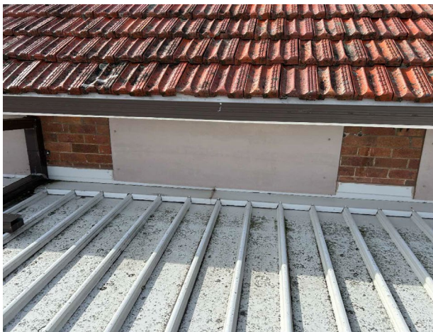
Line ID 34: External, Roof, ED Wing, West Side, Infill Panels, Fibre Cement Sheeting - None Suspected
