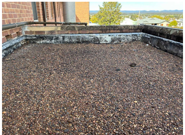
Line ID 35: External, Roof, Southeast Wing, Northwest Lower Roof Section, Waterproofing, Bituminous Membrane - Chrysotile Asbestos Detected
