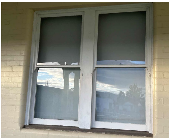
Line ID 5: External, GF, Cessnock House, East Wing, Windows, Window Caulking - No Asbestos Detected
