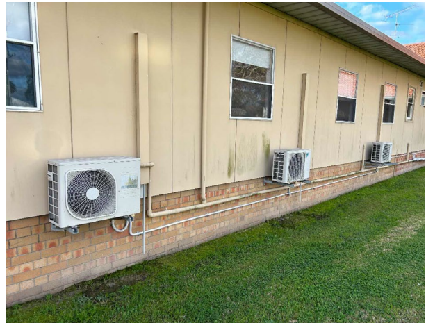
Line ID 45: External, GF, Pathology, East and West, AC Units, R410A Hydrofluorocarbon (HFC) - Non ODS Refrigerant
