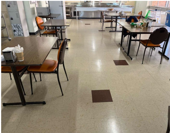
Line ID 11.1: Internal, GF, Kitchen, Cafeteria, Throughout, Vinyl Floor Tiles (white with brown specs) - Chrysotile Asbestos Detected
