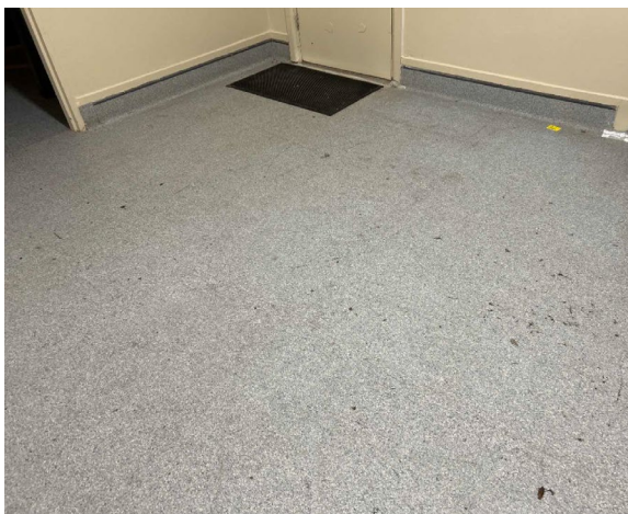
Line ID 11: Internal, GF, Cessnock House, East Wing, All Areas, Floor Below Vinyl Sheeting, Compressed Cement Sheeting - No Asbestos Detected
