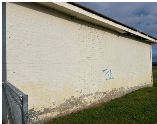
Line ID 34: External, GF, Old Mortuary, Walls, White Paint - Lead Detected (0.30% w/w)
