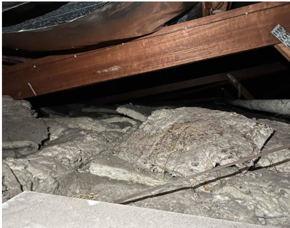
Line ID 17: Internal, GF, Storeroom Ceiling Space, Throughout, Insulation Batts - Suspected SMF
