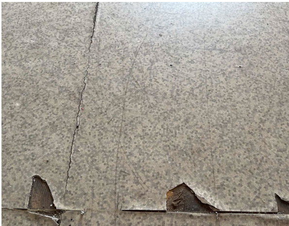
Line ID 41: Internal, GF, Palliative Care Storage Loading Dock, Floor Covering, Throughout, Vinyl Sheet (white) - No Asbestos Detected
