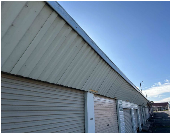
Line ID 13: External, GF, Workshops, All Areas, North and South Sections, Upper Walls, Profiled Cement Sheetting - Chrysotile Asbestos Detected
