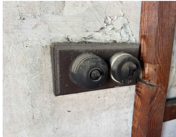
Line ID 17: Internal, GF, Old Mortuary, Various Throughout, Light Switches, Bakelite - Suspected Asbestos
