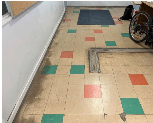
Line ID 7: Internal, GF, Storeroom, Main Foyer & Offices, Various Throughout, Vinyl Floor Tiles (red) - Chrysotile Asbestos Detected
