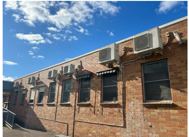
Line ID 169: External, GF, West Wing, South, East and West Sides, R410A Hydrofluorocarbon (HFC) - Non ODS Refrigerant
