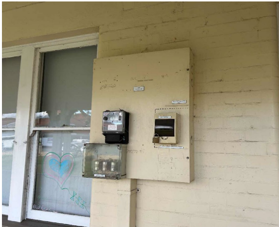
Line ID 3: External, GF, Cessnock House, East Wing, Veranda, Distribution Board, Electrical Components - Suspected Asbestos
