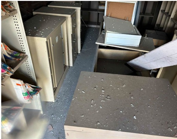
Line ID 46: Internal, GF, Workshops, Southern Section, Unit 1011, Debris on Surfaces, White Paint - Lead Detected (3.1% w/w)
