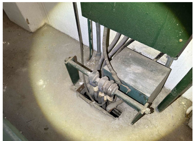
Line ID 100: Internal, L2, Lift Motor Room, Adjacent Motor, Wire Insulation, Woven Material - Suspected Asbestos
