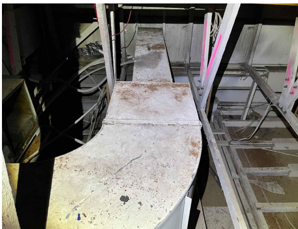
Line ID 143: Internal, GF, Central Wing, North Section, Ceiling Space, Ductwork, Throughout, Insulation Material - Suspected SMF
