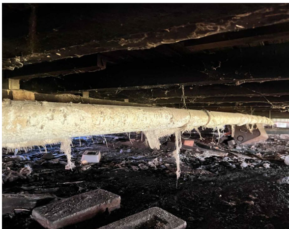
Line ID 8: External, GF, Workshops, All Areas, Central Section, Subfloor, Pipework, Lagging - Amosite Asbestos Detected
