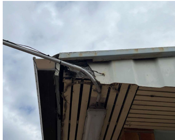
Line ID 2.1: External, GF, Mortuary, All Areas, Gable End, North & South, Moulded Fibre Cement - Chrysotile and Amosite Asbestos Detected
