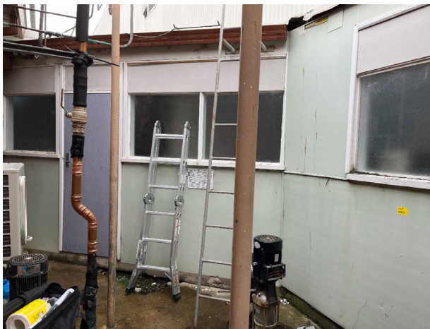
Line ID 2.1: External, GF, Central Wing, Central Courtyard, Wall Lining, Entry, Fibre Cement Sheeting - Chrysotile, Amosite and Crocidolite Asbestos Detected
