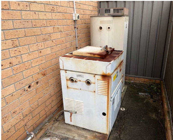
Line ID 32: External, GF, Cessnock House, West Wing, Hot Water Heater, Insulation Material - Suspected SMF
