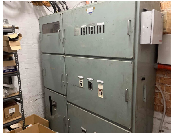
Line ID 30: Internal, GF, Main Switchboard Room, Electrical Distribution Board 1, Central, Compressed Bituminous Panel - Suspected Asbestos
