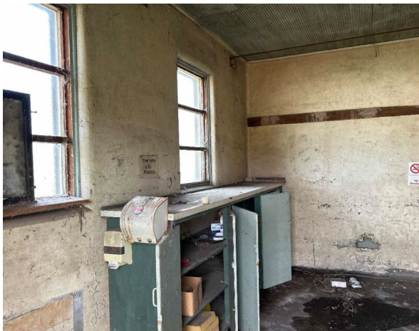
Line ID 43: Internal, GF, Old Mortuary, Walls, Cream Paint - Lead Detected (0.86% w/w)
