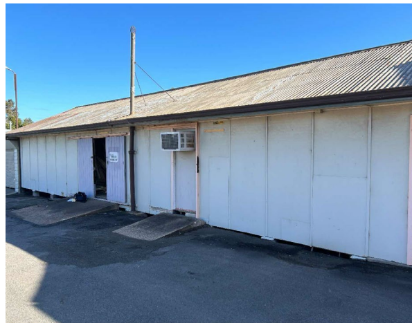
Line ID 5.1: External, GF, Workshops, All Areas, Central and North Sections, Walls, Fibre Cement Sheeting - Chrysotile, Amosite and Crocidolite Asbestos Detected
