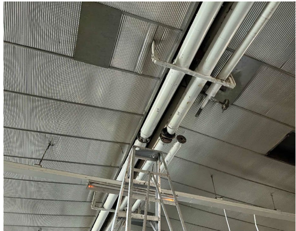
Line ID 23.1: Internal, GF, Laundry, Pipework, Central, Gasket Material - Chrysotile Asbestos Detected
