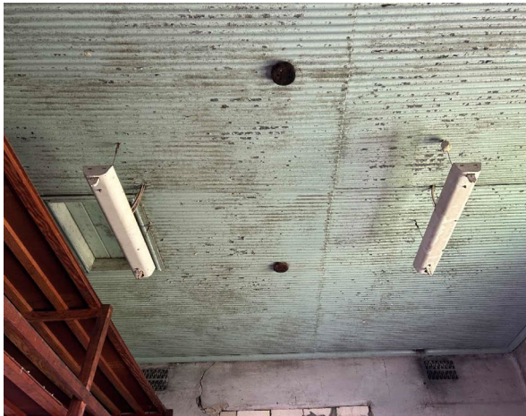
Line ID 54: Internal, GF, Old Mortuary, South Room, Light Fittings, Capacitor(s) - Suspected PCB
