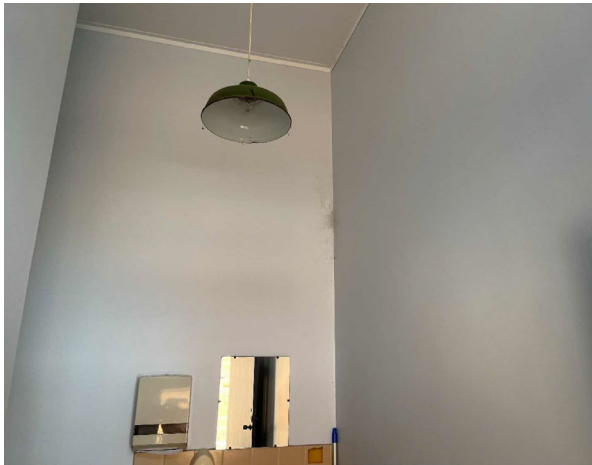
Line ID 53: Internal, GF, Room 1032, Toilet, Wall lining, Throughout, White Paint - Lead Detected (<0.005% w/w)
