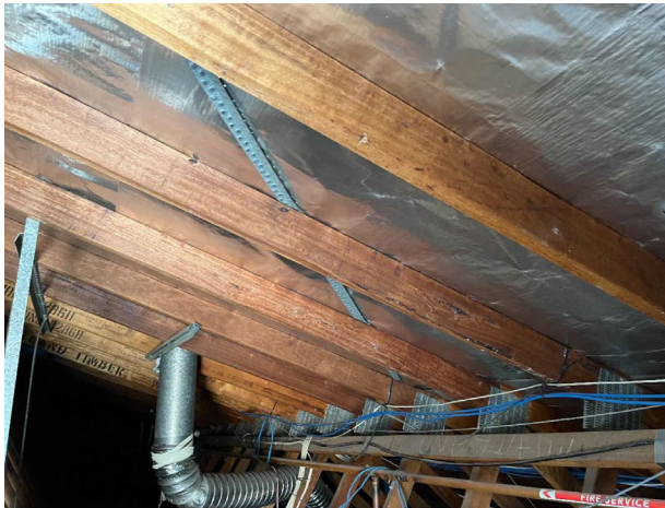
Line ID 157: Internal, GF, ED Wing, Ceiling Space, Sarking, Roof Lining, Insulation Material - Suspected SMF
