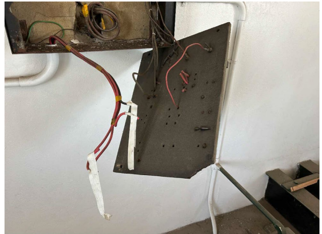
Line ID 102: Internal, L2, Lift Motor Room, Electrical Cabinet, Bituminous Backing Board - Suspected Asbestos
