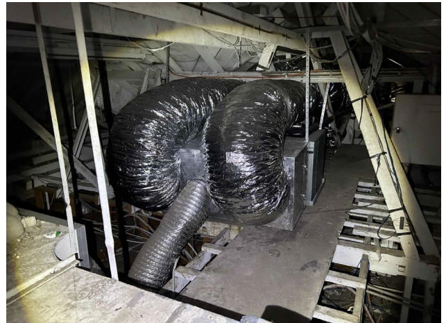
Line ID 135: Internal, GF, All Areas, Ceiling Space, Ductwork, Insulation Material - Suspected SMF
