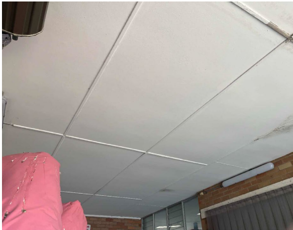
Line ID 40: Internal, GF, Palliative Care Storage Loading Dock, Ceiling lining, Throughout, Fibre Cement Sheeting - No Asbestos Detected
