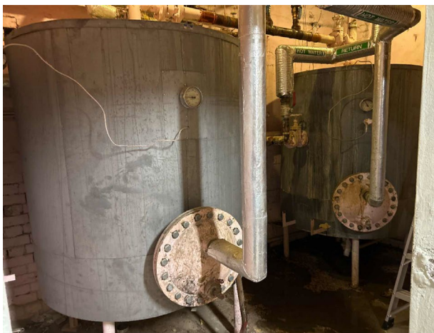
Line ID 52: Internal, GF, Central Wing, North Section, Plant Room 1073, Boilers, Insulation - Suspected Asbestos
