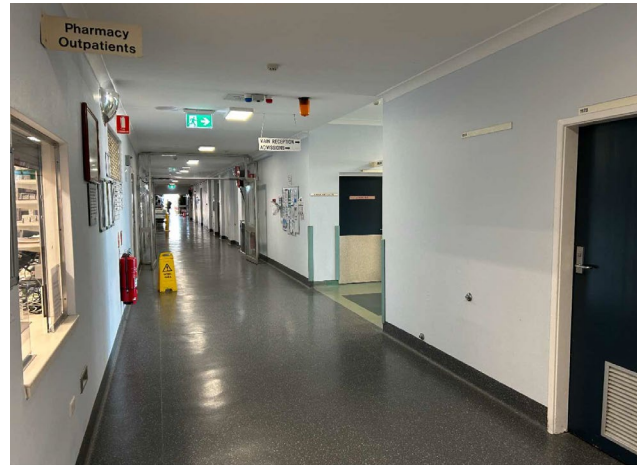
Line ID 112: Internal, GF, All Areas, Various Throughout, Walls, Light Purple Paint - Lead Detected (1.2 % w/w)
