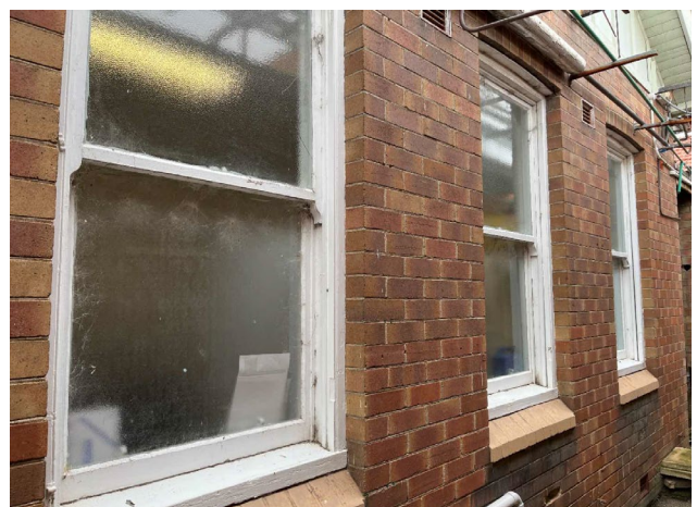
Line ID 106: External, GF, Central Wing, Central Courtyard, Windows & Frames, Throughout, White Paint - Lead Detected (1.8% w/w)
