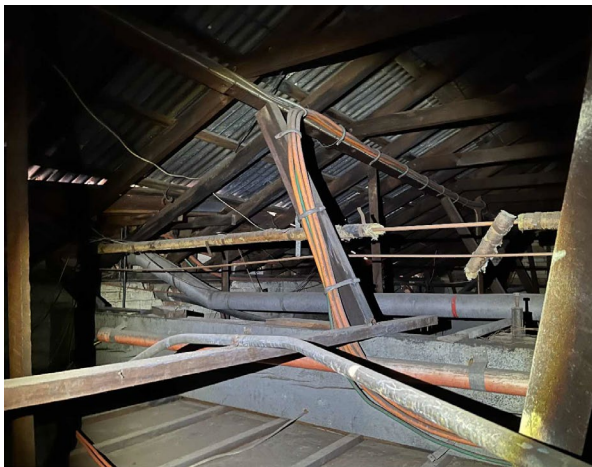
Line ID 32.1: Internal, GF, Main Workshop Area, Ceiling Space, Central, Lagging (metal encased material) - Suspected Asbestos
