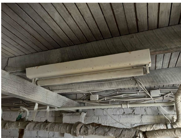
Line ID 161: Internal, GF, Southeast Wing, Southern Sub-Floor Area, Light Fittings, Capacitor(s) - Suspected PCB
