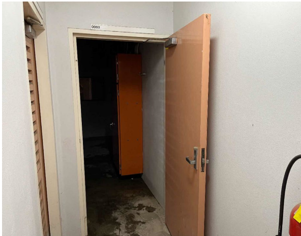
Line ID 22: Internal, Basement, Switchboard Room, 0003, Doors, Throughout, Brown (Light) Paint - Lead Detected (0.03% w/w)
