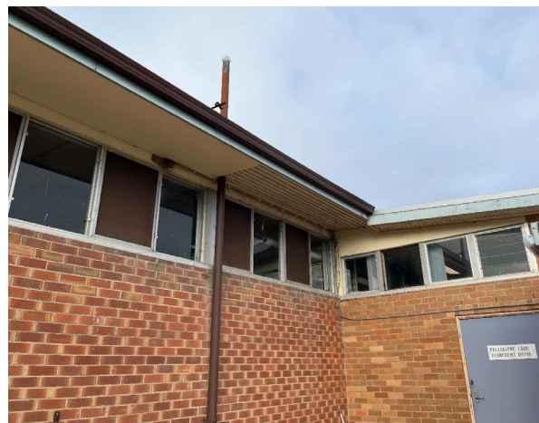
Line ID 4.1: External, GF, All Areas, Infill Panel, Above windows, Throughout, Fibre Cement Sheetting - Chrysotile Asbestos Detected
