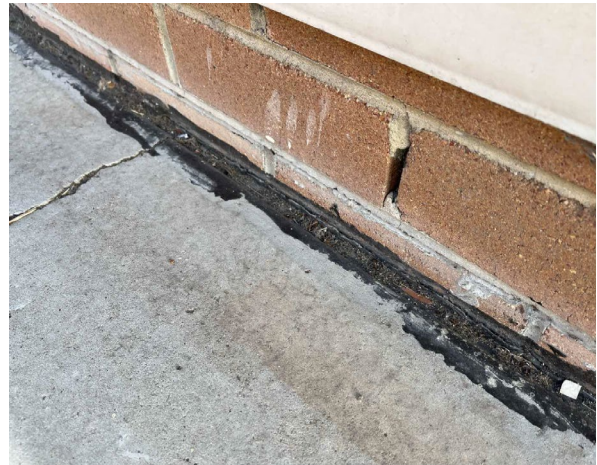
Line ID 7: External, GF, All Areas, Walkway Between Palliative Storage and Emergency, Below Window, Construction Joint Mastic - No Asbestos Detected
