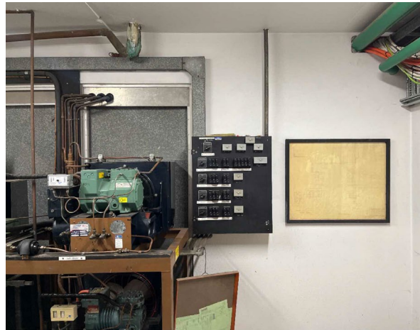
Line ID 17: Internal, Basement, Switchboard Room, 0003, Electrical Distribution Board, Southwest, Compressed Bituminous Panel - Suspected Asbestos
