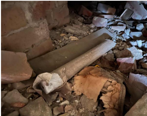
Line ID 10.1: External, GF, Subfloor Entrance, Pipework Lagging, Throughout, Lagging Debris - Amosite Asbestos Detected
