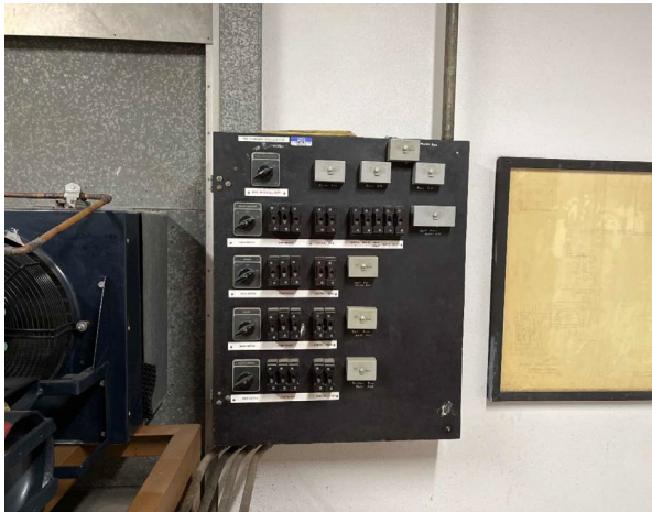
Line ID 16: Internal, Basement, Switchboard Room, 0003, Electrical Distribution Board, Southwest, Internal Components - Suspected Asbestos
