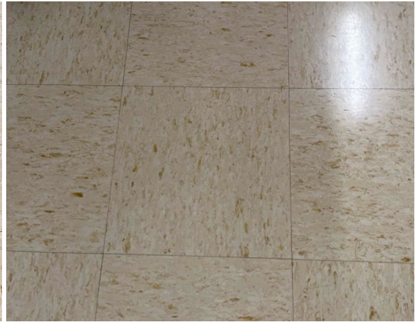
Line ID 11: Internal, GF, Kitchen, Cafeteria, Throughout, Vinyl Floor Tiles (white with brown specs) - Chrysotile Asbestos Detected
