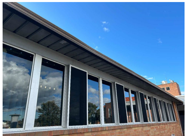
Line ID 11: External, GF, Central Wing, South Side, Infill Panels Above Windows, Fibre Cement Sheetting - Chrysotile Asbestos Detected
