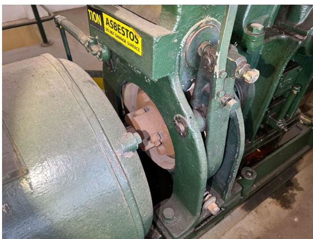
Line ID 105: Internal, L2, Lift Motor Room, Lift Motor, Friction Pads - Suspected Asbestos
