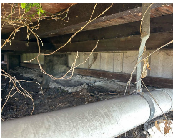
Line ID 10: External, GF, Workshops, All Areas, Central Section, Subfloor, South Wall, Profiled Cement Sheetting - Chrysotile Asbestos Detected
