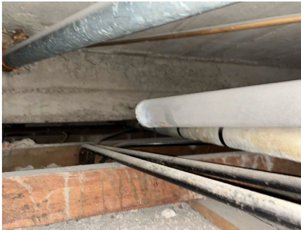
Line ID 80: Internal, GF, Southeast Wing, Ceiling Space, Throughout, Lagging - Amosite Asbestos Detected
