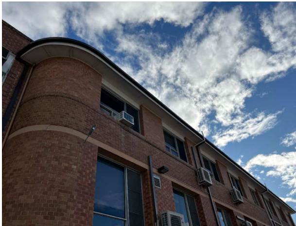
Line ID 27: External, L1, Southeast Wing, Throughout, Eaves, Fibre Cement Sheeting - Chrysotile Asbestos Detected
