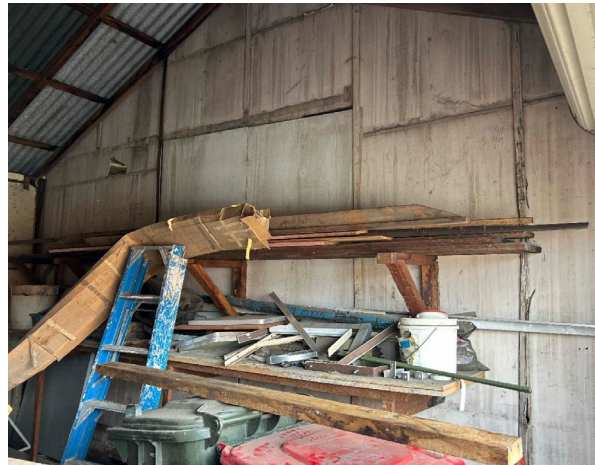
Line ID 22: Internal, GF, Workshops, Central Section, North Store Room, North and South, Walls, Fibre Cement Sheetting - Chrysotile, Amosite and Crocidolite Asbestos Detected
