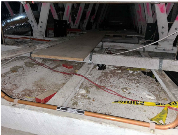
Line ID 122: Internal, GF, Central Wing, North Section, Ceiling Space, Throughout, Dust - Lead Detected (49mg/kg)
