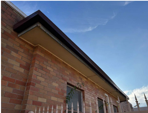
Line ID 24: External, GF, West Wing, South Side, Eaves, Fibre Cement Sheetting - Chrysotile Asbestos Detected
