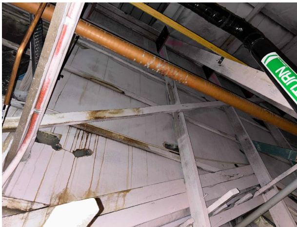
Line ID 44: Internal, GF, Central Wing, North Section, Ceiling Space, South and East Sides, Walls, Fibre Cement Sheeting – Suspected Asbestos
