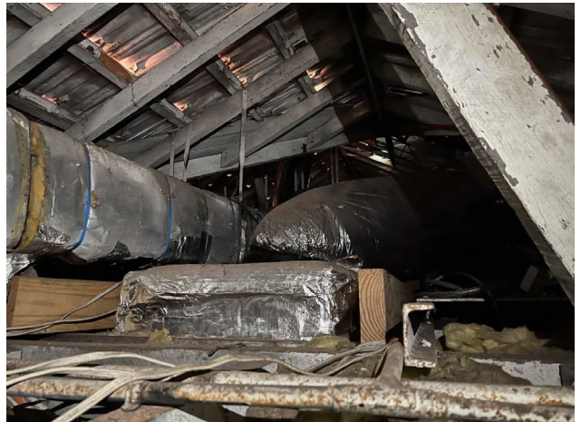
Line ID 148: Internal, GF, Central Wing, North Section, Plant Room 1119, Ceiling Space, Insulation Batts, Insulation Material - Suspected SMF
