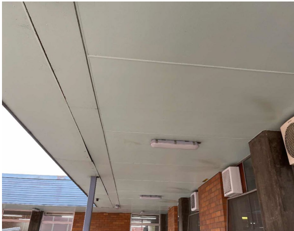
Line ID 1: External, GF, All Areas, Awning, Southeast Verandah, Fibre Cement Sheetting - Chrysotile Asbestos Detected
