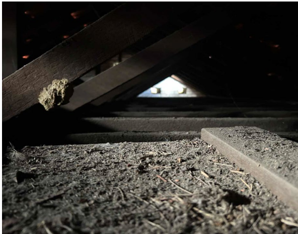
Line ID 48: Internal, GF, Old Mortuary, Ceiling Space, Dust - Lead Detected (290 mg/kg)
