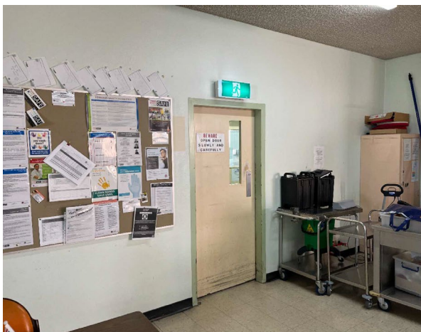
Line ID 20.1: Internal, GF, Kitchen, Door Frames, Throughout, Green (Light) Paint - Lead Detected (0.099% w/w)
