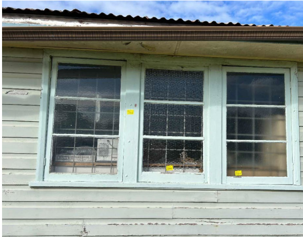
Line ID 37: External, GF, Workshops, All Areas, Central Section, West, Window Frames, White Paint - Lead Detected (0.24% w/w)
