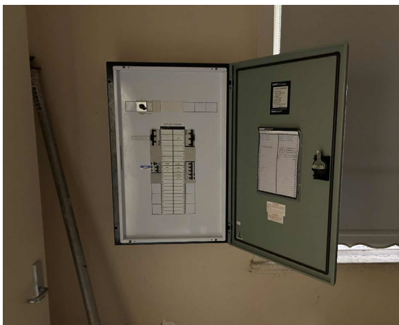
Line ID 16: Internal, GF, Cessnock House, East Wing, Southeast Room, Distribution Board, Electrical Components - Suspected Asbestos
