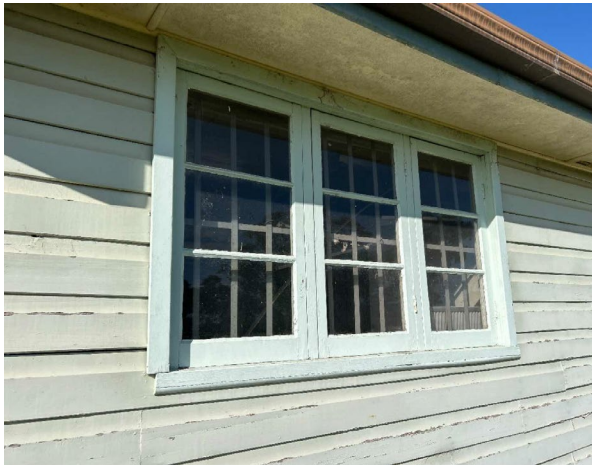
Line ID 12: External, GF, Workshops, All Areas, Central Section, West Windows, Thick Window Caulking - No Asbestos Detected
