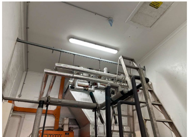
Line ID 150: Internal, GF, Central Wing, North Section, Plant Room 1119, Pipework, Insulation Material - Suspected SMF
