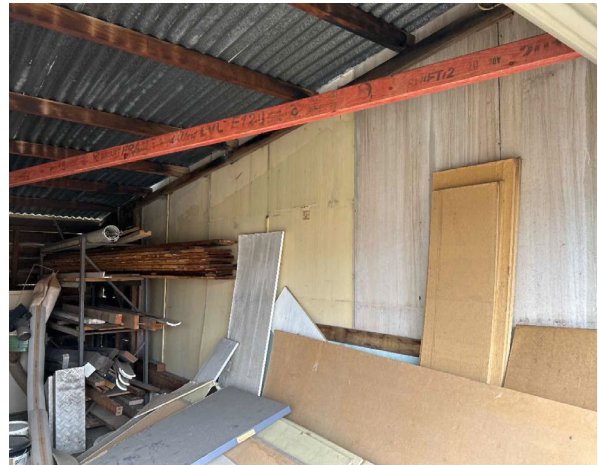
Line ID 26: Internal, GF, Workshops, Southern Section, Northern Unit, North, Wall, Fibre Cement Sheeting - Chrysotile, Amosite and Crocidolite Asbestos Detected
