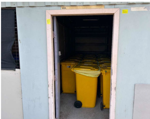
Line ID 39: External, GF, Workshops, All Areas, North Sections, Northeast, Door Frame, Cream Paint - Lead Detected (0.12% w/w)
