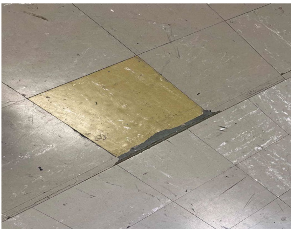
Line ID 21: Internal, GF, Laundry, Floor Covering, Various Throughout, Vinyl Floor Tiles (khaki green with white specs) - Chrysotile Asbestos Detected
