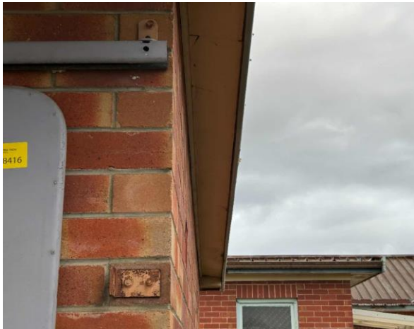
Line ID 4: External, GF, Dangerous Goods Store, North and South, Eaves, Fibre Cement Sheeting - Chrysotile, Amosite and Crocidolite Asbestos Detected
