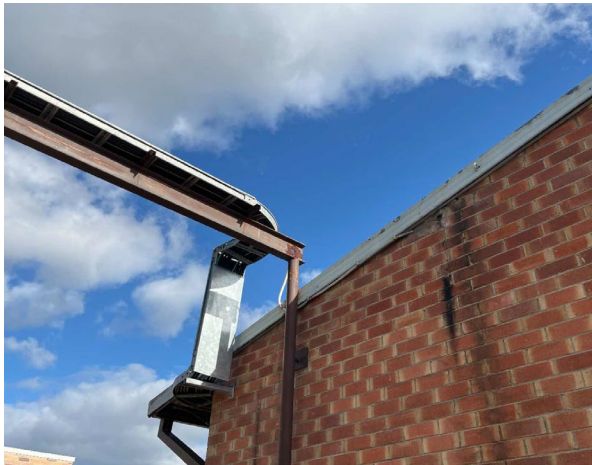
Line ID 12: External, GF, Storeroom Driveway, Metal Works, Various Throughout, Blue (Light) Paint - Lead Detected (0.10% w/w)
