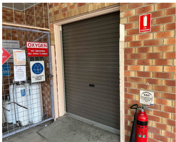
Line ID 10.1: External, GF, Mortuary, All Areas, Door & Frames, Throughout, Pink (Light) Paint - Lead Detected (0.18% w/w)
