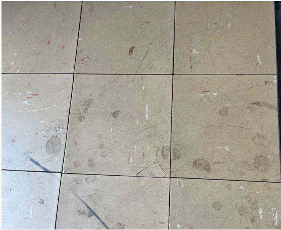
Line ID 5.1: Internal, GF, Storeroom, Main Foyer & Offices, Throughout, Vinyl Floor Tiles (cream with white specs) - Chrysotile Asbestos Detected
