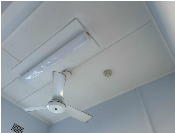
Line ID 86: Internal, GF, Southeast Wing, Rooms 1201, 1202, and 1203, Ceiling, Fibre Cement Sheeting - Chrysotile Asbestos Detected
