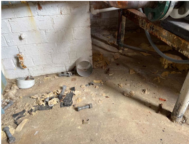
Line ID 141: Internal, GF, Central Wing, Day Surgery/Recovery, Plant Room, Pipework Debris, Insulation Material - Suspected SMF
