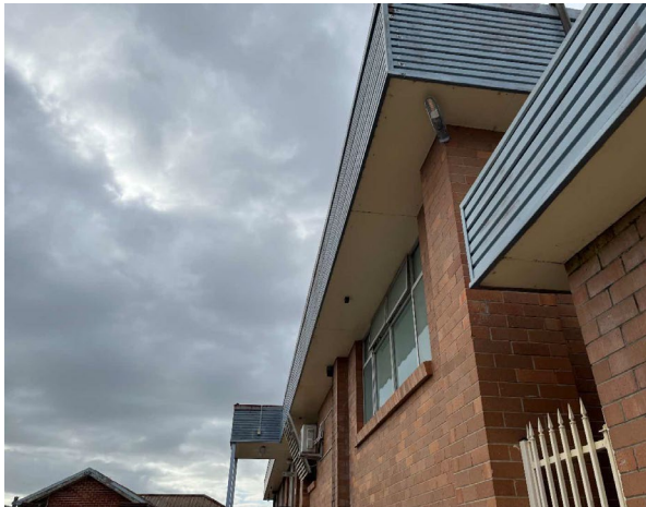
Line ID 2: External, GF, All Areas, Eaves, Throughout, Fibre Cement Sheetting - Chrysotile Asbestos Detected
