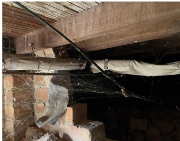
Line ID 9: External, GF, Subfloor Entrance, Pipework Lagging, Throughout, Lagging - Amosite Asbestos Detected
