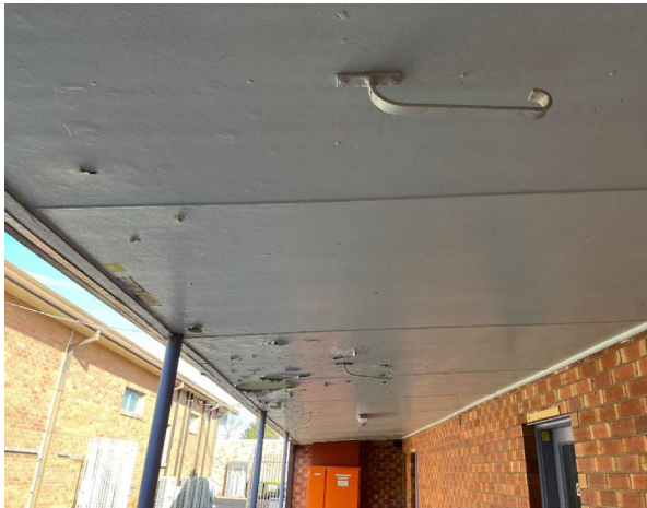
Line ID 48.1: External, GF, All Areas, Ceiling lining, Adjacent Clinical Information Department Entrance, White Paint - Lead Detected (0.14% w/w)
