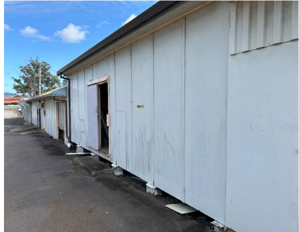
Line ID 38: External, GF, Workshops, All Areas, North and Central Sections, Walls, White Paint - Lead Detected (0.18% w/w)
