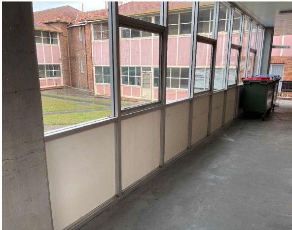
Line ID 5: External, GF, All Areas, Metal Windows, Throughout, Window Caulking - Chrysotile Asbestos Detected
