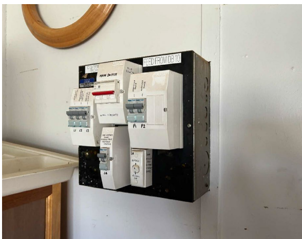
Line ID 20: Internal, GF, Workshops, Central Section, Central Office, Northeast, Bituminous Backing Board - Suspected Asbestos
