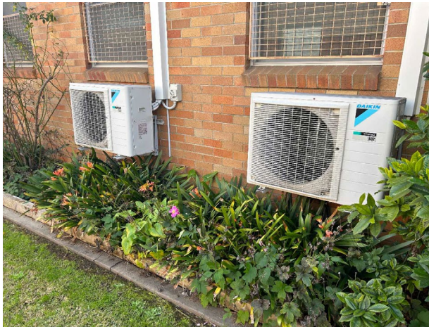
Line ID 168: External, GF, West Wing, South Side, R32 Refrigerant - Non ODS Refrigerant
