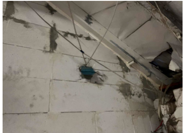
Line ID 154: Internal, GF, Central Wing, Ward A & B, Ceiling Space, Pillow insulation, Penetrations adjacent ladder, Insulation Material - Suspected SMF
