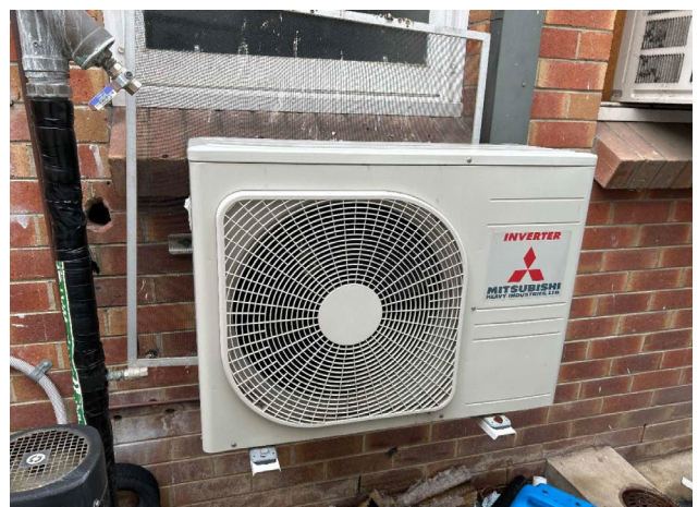
Line ID 162: External, GF, Central Wing, Central Courtyard, AC Unit, R410A Hydrofluorocarbon (HFC) - Non ODS Refrigerant
