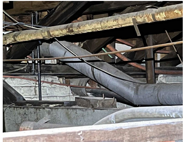
Line ID 32: Internal, GF, Main Workshop Area, Ceiling Space, Central, Lagging (metal encased material) - Suspected Asbestos
