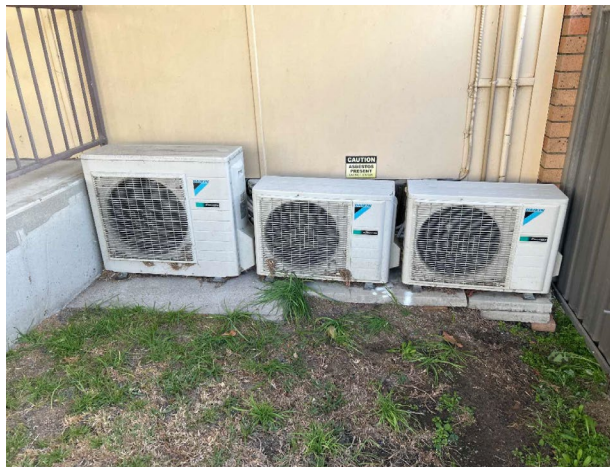
Line ID 41: External, GF, Cessnock House, East Wing, North, AC Units, R410A Hydrofluorocarbon (HFC) - Non ODS Refrigerant
