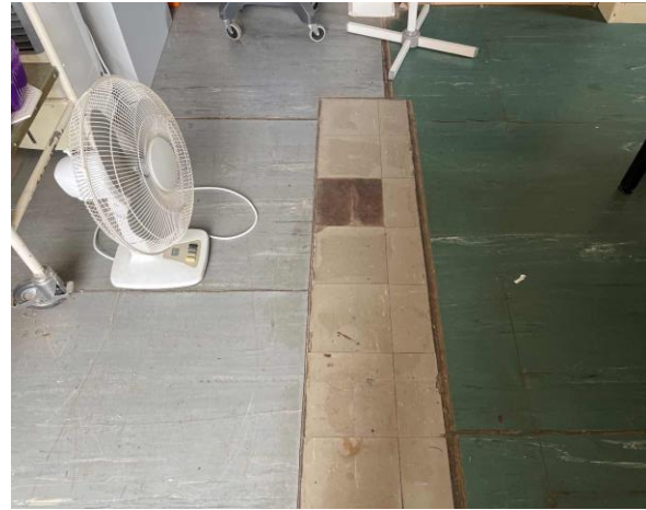
Line ID 14.1: Internal, GF, Dining/Laundry, Floor Covering, Various Throughout, Vinyl Floor Tiles - Chrysotile Asbestos Detected
