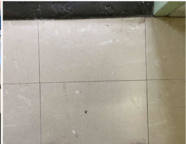
Line ID 12: Internal, GF, Kitchen, Room 1010 Cleaners Cupboard, Throughout, Vinyl Floor Tiles (white) - Chrysotile Asbestos Detected
