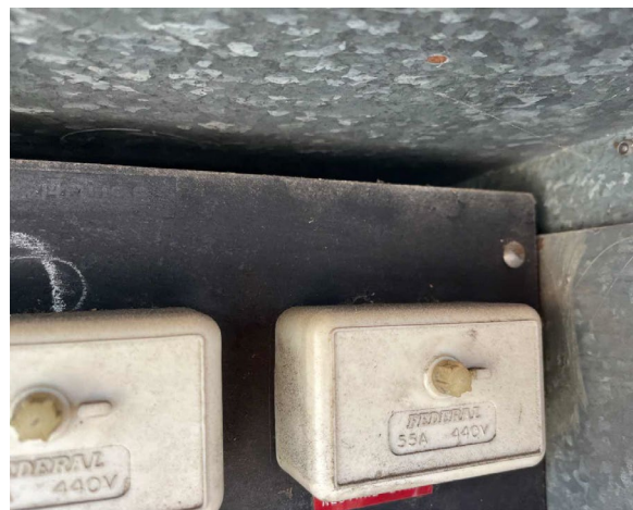
Line ID 3.1: External, GF, Storeroom Driveway, Electrical Distribution Board, Northern Boundary, Compressed Bituminous Panel - Suspected Asbestos
