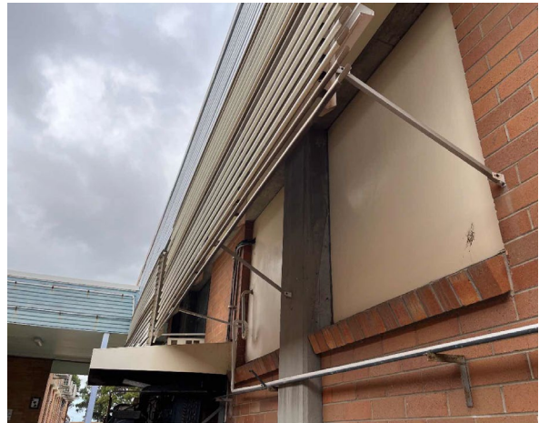
Line ID 3: External, GF, All Areas, Infill Panels, Adjacent Air Conditioning Refrigerator Pump, Fibre Cement Sheet - Chrysotile Asbestos Detected
