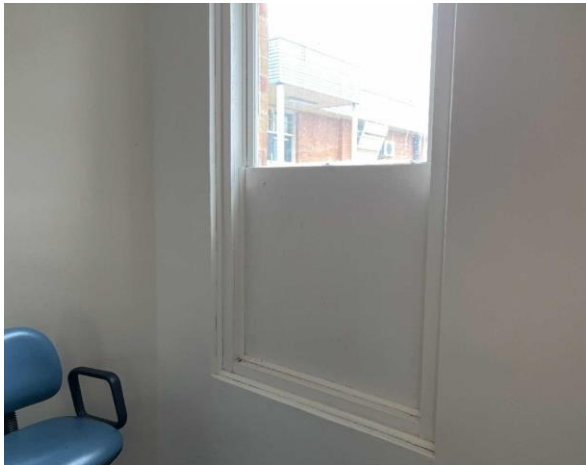
Line ID 15: Internal, GF, Dining/Laundry, Infill panel, Below Window, Fibre Cement Sheet - Chrysotile Asbestos Detected
