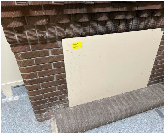
Line ID 13: Internal, GF, Cessnock House, East Wing, Fireplace, Infill Panel, Compressed Cement Sheet - Chrysotile Asbestos Detected
