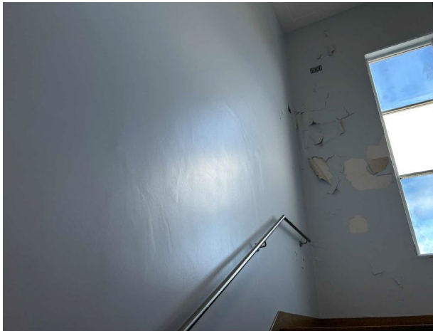
Line ID 118: Internal, GF, Southeast Wing, All Areas, Walls, Light Purple Paint - Lead Detected (1.2 % w/w)
