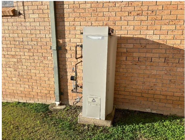
Line ID 33: External, GF, Cessnock House, West Wing, South, Water Heater, Insulation Material - Suspected SMF
