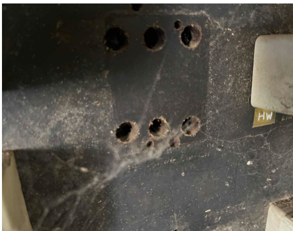
Line ID 23.2: Internal, GF, Workshops, Northern Section, Electrical Distribution Board 19 - Incinerator, Compressed Bituminous Panel - Suspected Asbestos
