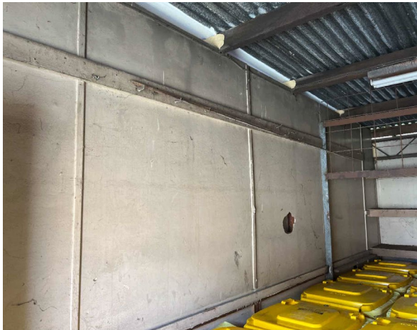
Line ID 25.1: Internal, GF, Workshops, Northern Section, Wall Lining, Fibre Cement Sheeting - Chrysotile, Amosite and Crocidolite Asbestos Detected
