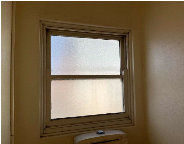
Line ID 14: Internal, GF, Storeroom, Windows & Frames, Various Throughout, White Paint - Lead Detected (0.21% w/w)
