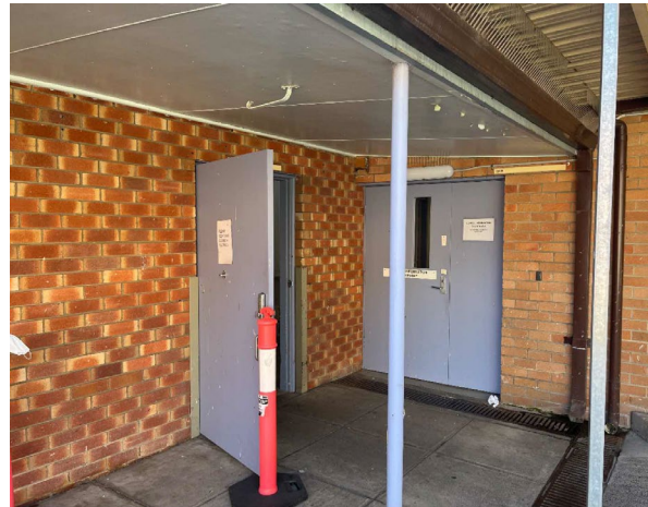
Line ID 49: External, GF, All Areas, Door & Frames, Throughout, Purple (Light) Paint - Lead Detected (0.04% w/w)
