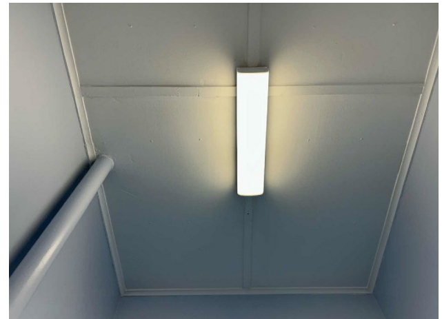
Line ID 86.1: Internal, GF, Southeast Wing, Rooms 1201, 1202, and 1203, Ceiling, Fibre Cement Sheeting - Chrysotile Asbestos Detected
