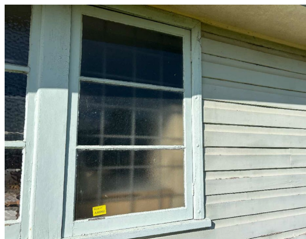
Line ID 11: External, GF, Workshops, All Areas, Central Section, West Windows, Thin Window Caulking - No Asbestos Detected
