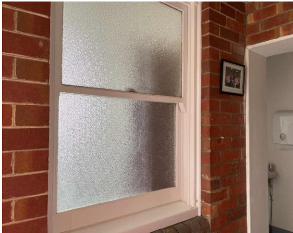
Line ID 23: Internal, GF, All Areas, Windows & frames, Throughout, White Paint - Lead Detected (0.34% w/w)
