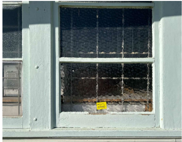
Line ID 12.1: External, GF, Workshops, All Areas, Central Section, West Windows, Thick Window Caulking - No Asbestos Detected
