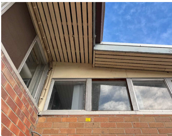
Line ID 4: External, GF, All Areas, Infill Panel, Above windows, Throughout, Fibre Cement Sheetting - Chrysotile Asbestos Detected
