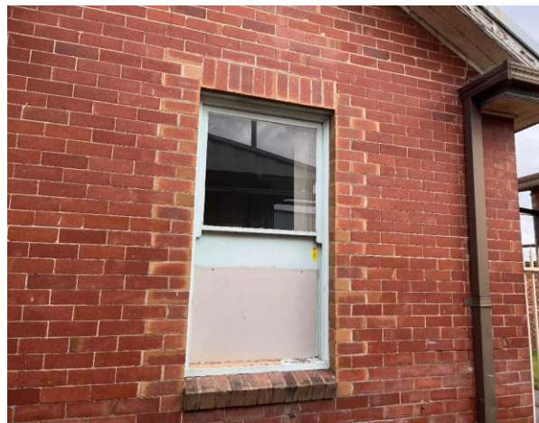
Line ID 2.2: External, GF, All Areas, Infill Panels, Below Windows, Fibre Cement Sheet - Chrysotile, Amosite and Crocidolite Asbestos Detected
