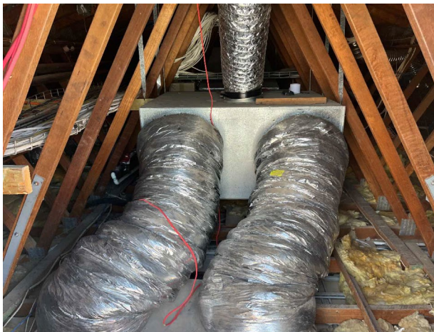
Line ID 155: Internal, GF, ED Wing, Ceiling Space, Ductwork, Various Throughout, Insulation Batts - Suspected SMF
