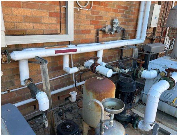
Line ID 8: External, GF, Central Wing, Northern Boiler Area, Metal Encased Pipework, Lagging - Suspected Asbestos
