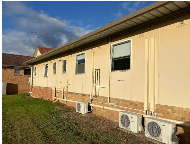
Line ID 10: External, GF, Pathology, West Wall, Fibre Cement Sheeting - Chrysotile Asbestos Detected
