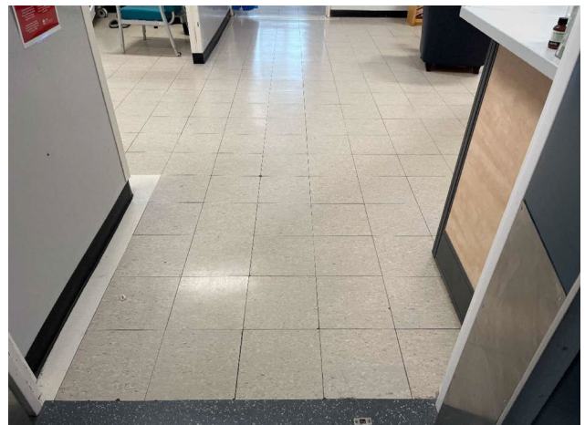
Line ID 78: Internal, GF, Central Wing, Ward B, Rooms 1174, 1176 & 1177, Floor Covering, Vinyl Floor Tiles (white with grey specks) - Chrysotile Asbestos Detected
