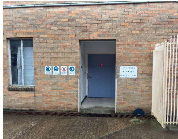
Line ID 12.1: External, GF, Workshop Entrance, Wall Lining, Fibre Cement Sheeting - Chrysotile Asbestos Detected
