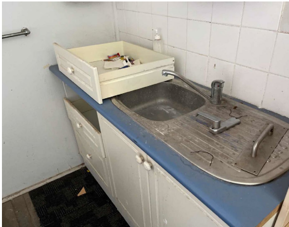
Line ID 21.1: Internal, GF, Workshops, Central Section, Kitchenette, Under Sink, Sink Pad (no access), Bituminous Material - Chrysotile Asbestos Detected
