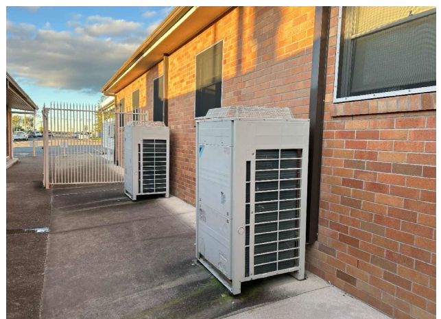
Line ID 167: External, GF, ED Wing, North Side, AC Unit, R410A Hydrofluorocarbon (HFC) - Non ODS Refrigerant
