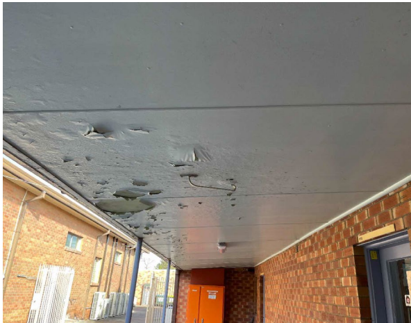
Line ID 1: External, GF, Adjacent Clinical Information Department Entrance, Awning, Fibre Cement Sheetting - Chrysotile Asbestos Detected
