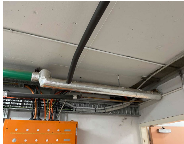
Line ID 25: Internal, Basement, Switchboard Room, 0003, Pipework, Throughout, Insulation Material - Suspected SMF
