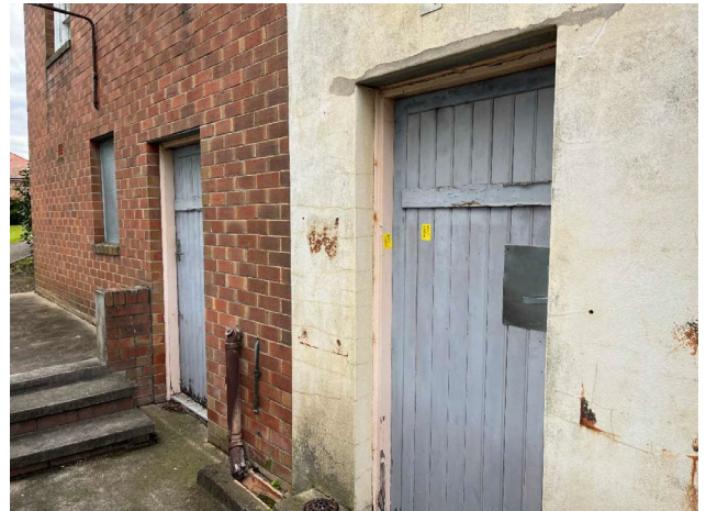
Line ID 109: External, GF, Southeast Wing, Door & Frames, Various Throughout, Pink (Light) Paint - Lead Detected (0.02% w/w)
