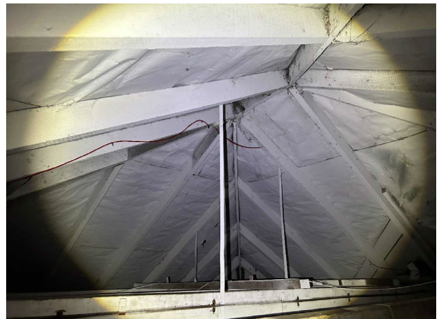
Line ID 137: Internal, GF, All Areas, Ceiling Space, Throughout, Sarking Insulation - Suspected SMF
