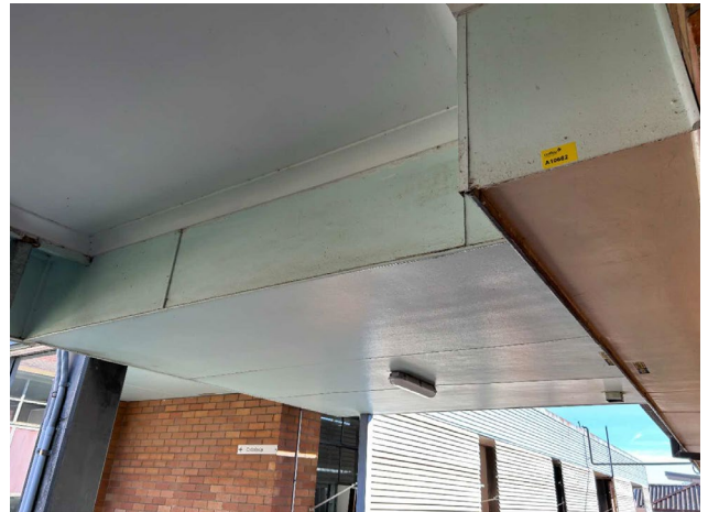
Line ID 25: External, GF, West Wing, Western Covered Area Adjacent Kitchen, Awning and Infill Panels, Fibre Cement Sheetting - Chrysotile Asbestos Detected
