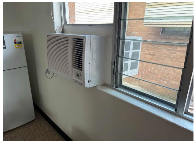
Line ID 173: Internal, GF, Central Wing, Ward A, Staff Room 1118, AC Unit, Unknown Refrigerant - Suspected ODS
