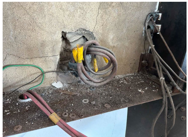
Line ID 104: Internal, L2, Lift Motor Room, Electrical Cabinet, Wire Insulation, Woven Material - Suspected Asbestos
