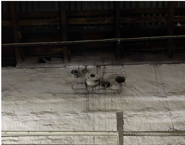
Line ID 39: Internal, GF, Painters Shop, Pipework Penetration, Northeast Adjacent Generator, Lagging - Amosite Asbestos Detected
