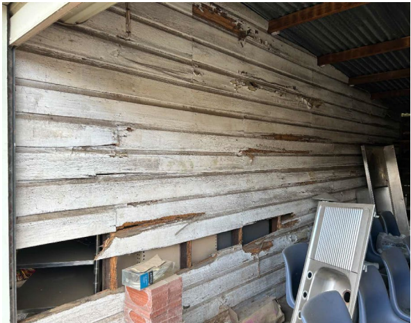
Line ID 47: Internal, GF, Workshops, Southern Section, Various Timber Walls, White Paint - Lead Detected (0.18% w/w)
