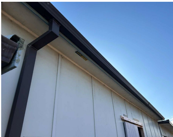
Line ID 3: External, GF, Workshops, All Areas, Central and North Sections, Eaves, Fibre Cement Sheeting - Chrysotile, Amosite and Crocidolite Asbestos Detected
