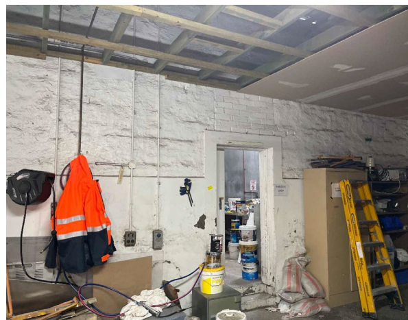
Line ID 52: Internal, GF, Painters Shop, Wall Lining, Throughout, White Paint - Lead Detected (0.04% w/w)
